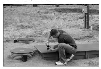
**WARNING:** If lid bolts are missing, replace them with spares. If you have no spare lid bolts, fasten the lid with a self-tapping screw, and immediately call your Dealer for replacement bolts. If the lid is unbolted or if the lid or riser are damaged, be sure to securely block access to the tank opening before leaving the site. Open tanks are hazardous, and children or adults who try to enter them may be seriously injured, asphyxiated, or drowned.
