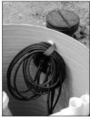
Splice box mounted in discharge access riser. Watertight connectors used.
