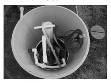
☐ Float assembly mounted in Biotube® vault.
