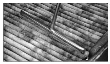
If you need to clean the sheets, <u>remove the RSV</u> so that solids can freely drain back to the tank. Then clean the sheets one by one with the
