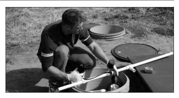
Raise the bottom float to stop the alarm. A yellow LED should light up.
