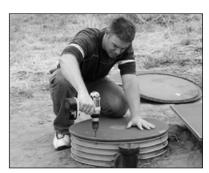
WARNING: If lid bolts are missing, replace them with spares. If you have no spare lid bolts, fasten the lid with a self-tapping screw, and immediately call your Dealer for replacement bolts. If the lid is unbolted or if the lid or riser are damaged, be sure to securely block access to the tank opening before leaving the site. Open tanks are hazardous, and children or adults who try to enter them may be seriously injured, asphyxiated or drowned.
