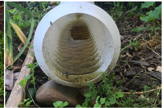
Plastic downspout extensions holding water
