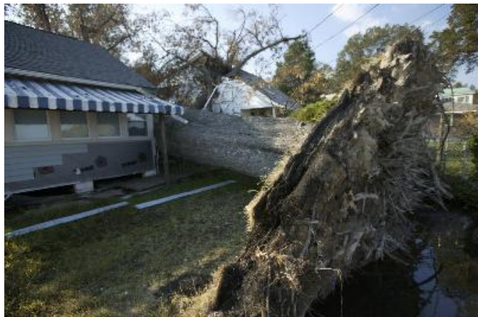
Hurricane damage in Colonial Beach. Winds from Hurricane Isabel in 2003 downed trees, cut power lines, and severed water distribution pipe throughout Virginia.
