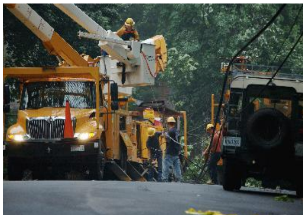
Contractors work to repair a power line that was taken down by a tree in Northern Virginia after a summer storm.
