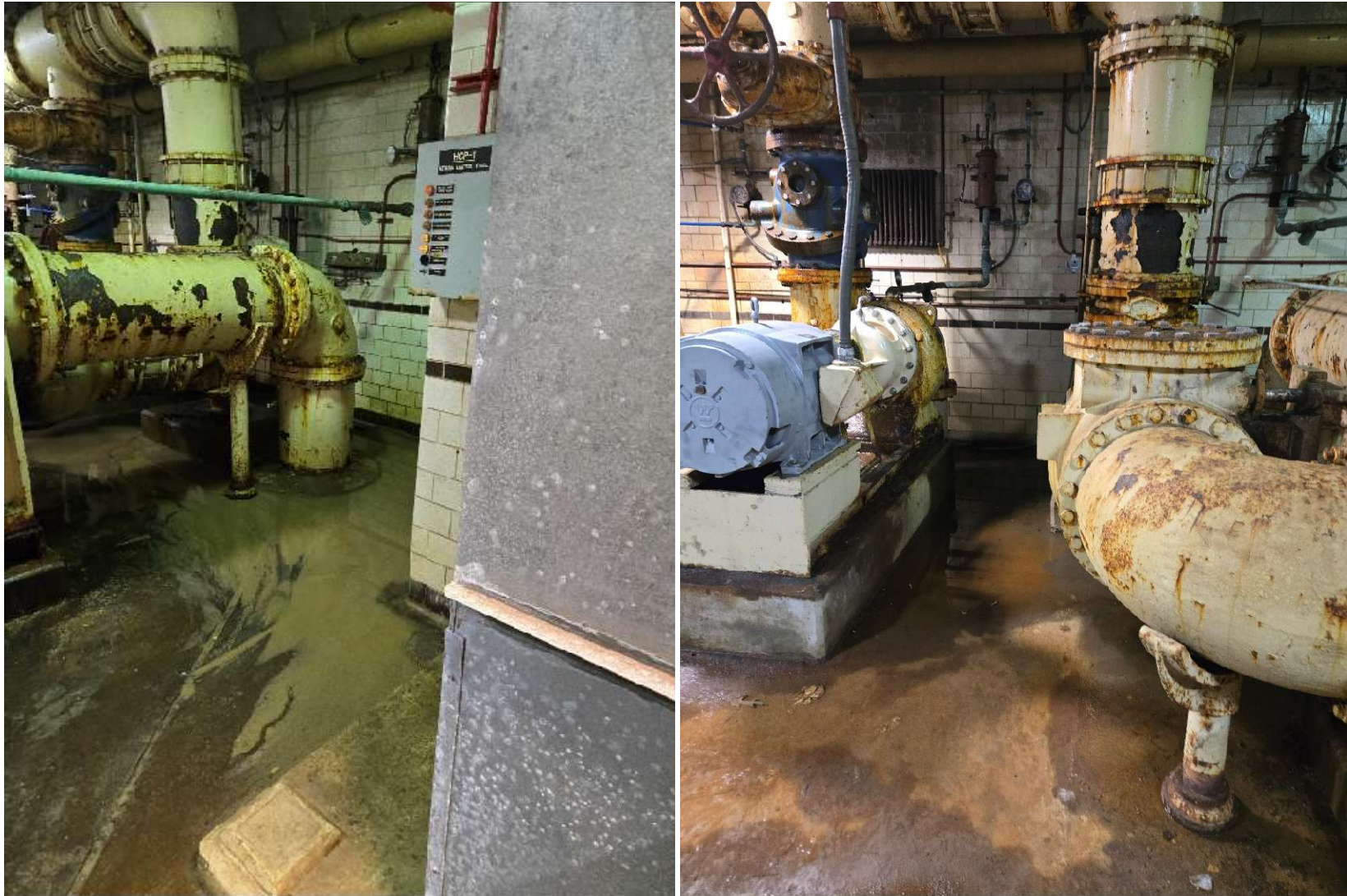
Figure 19. Backwash waste area (2025); (2026)
