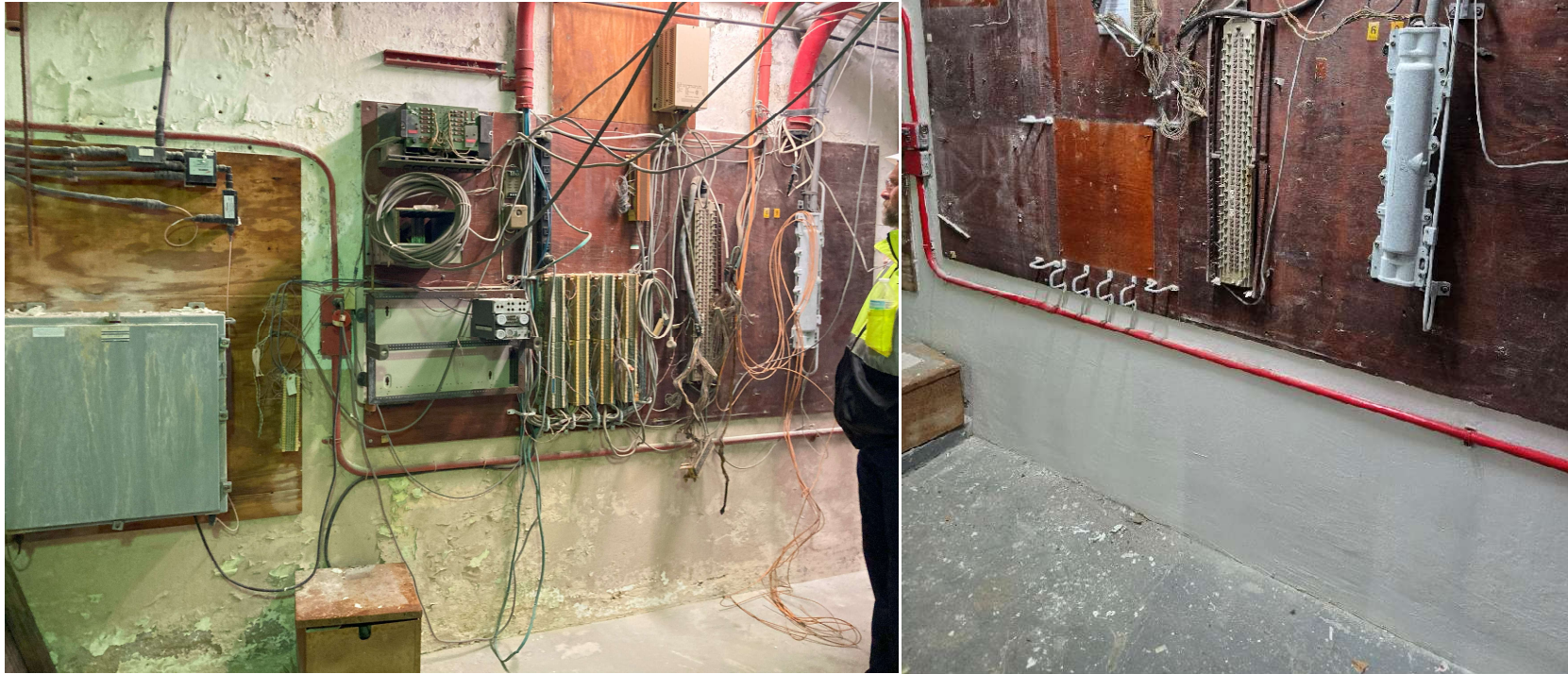
Figure 15. Obsolete equipment abandoned in place (2025), Wiring removed as much as possible (2026)
