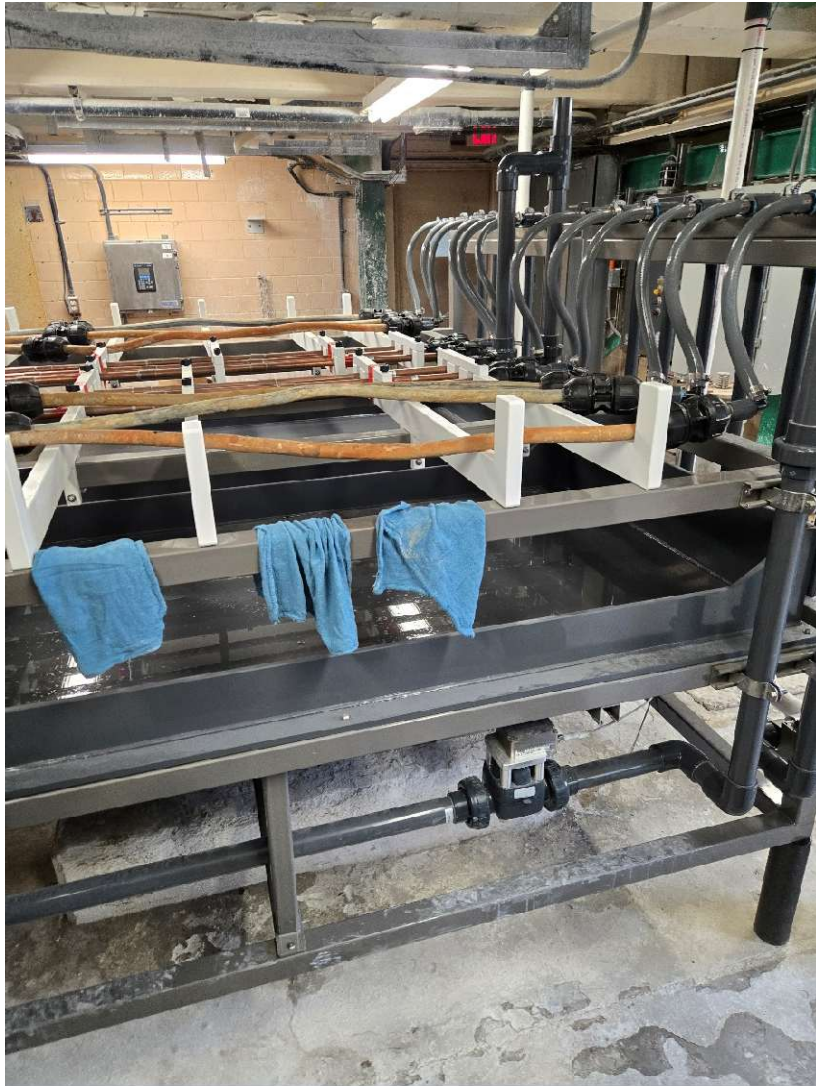
Figure 26. Pipe loop installation
