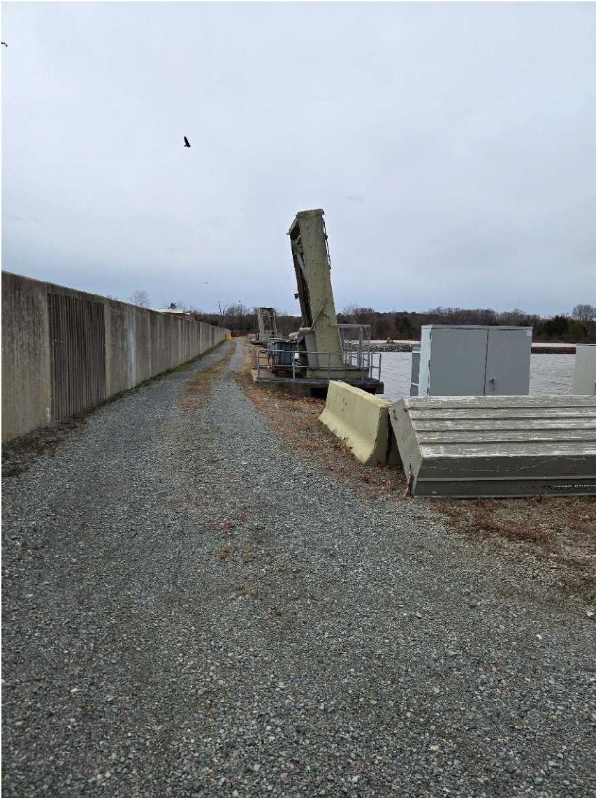
Figure 5. Pre-sed traveling screens
