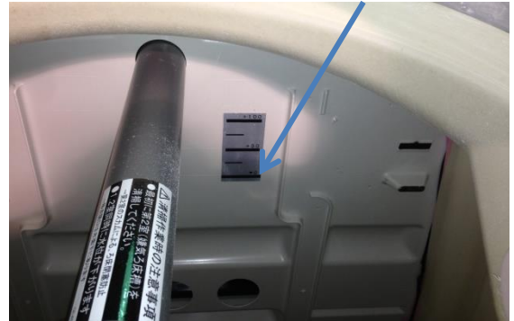
Low water line in sedimentation chamber
