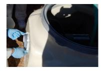
Seal around inlet and outlet tank fittings using a sealant that meets ASTM C990-96 standards
