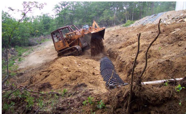
Figure: 6-22. Compaction during construction of this shallow system on a 30% slope may reduce the lifespan of the system. (Photo by Tom Saxton)
