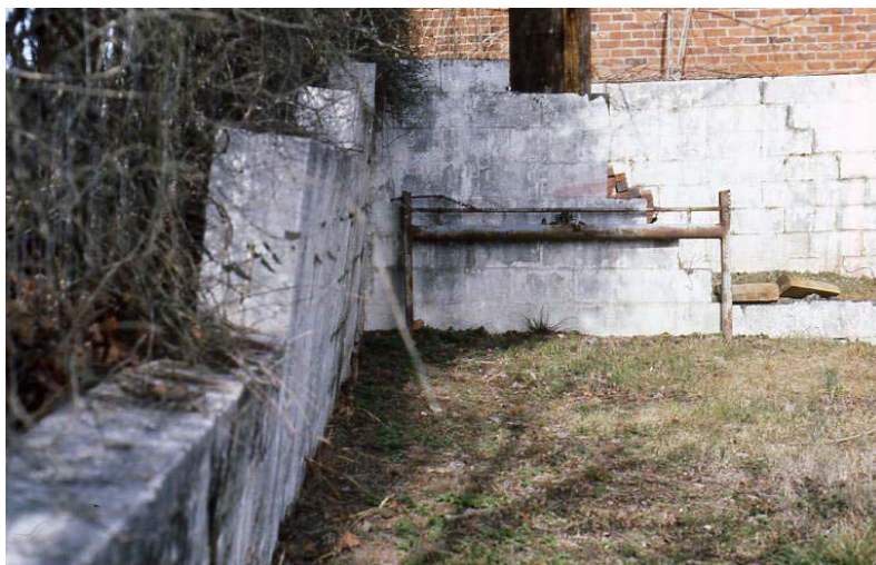
Figure: 6-19. This wall is collapsing due to an unstable footing in shrink-swell soils. (Photo by Tom Saxton)
