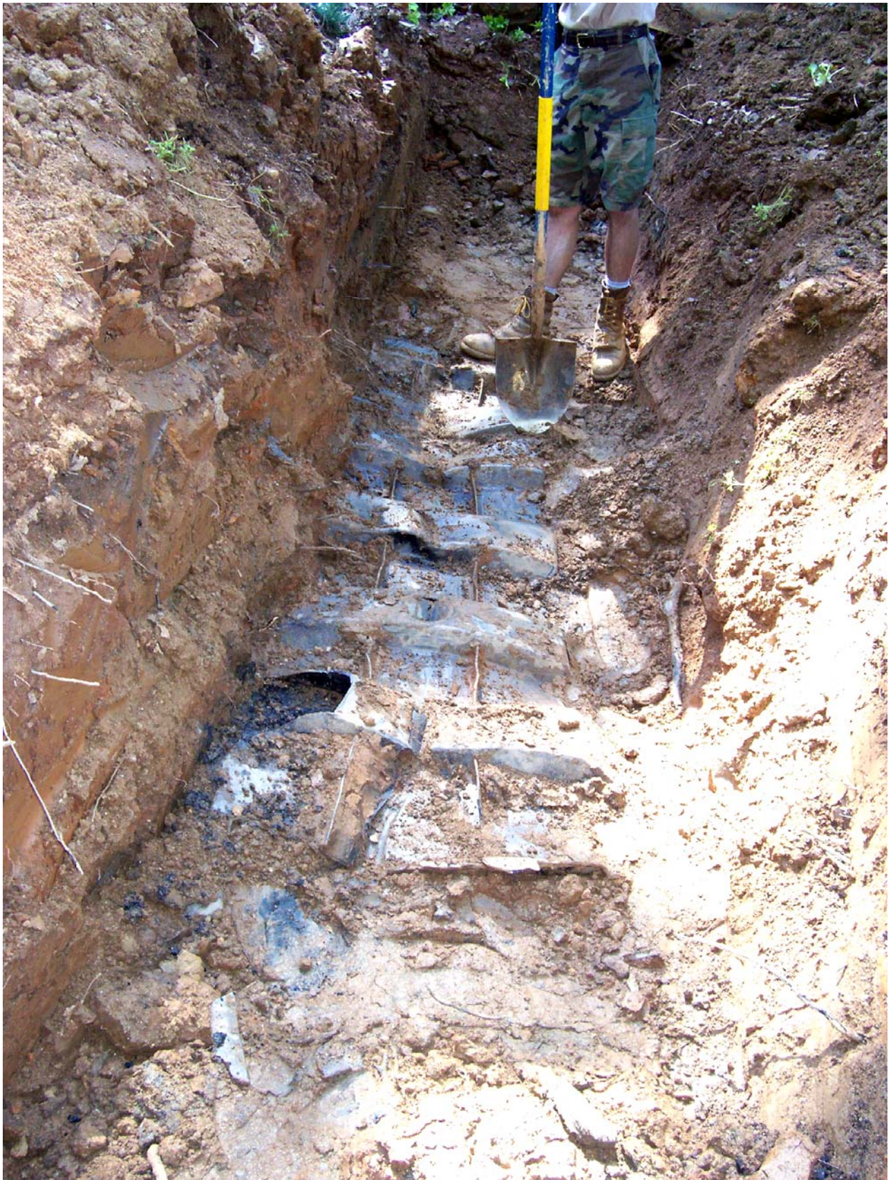
Figure: 7-20. This chamber system was apparently crushed when the trenches were filled. (Photo by Todd Fowler, EH Supervisor)
