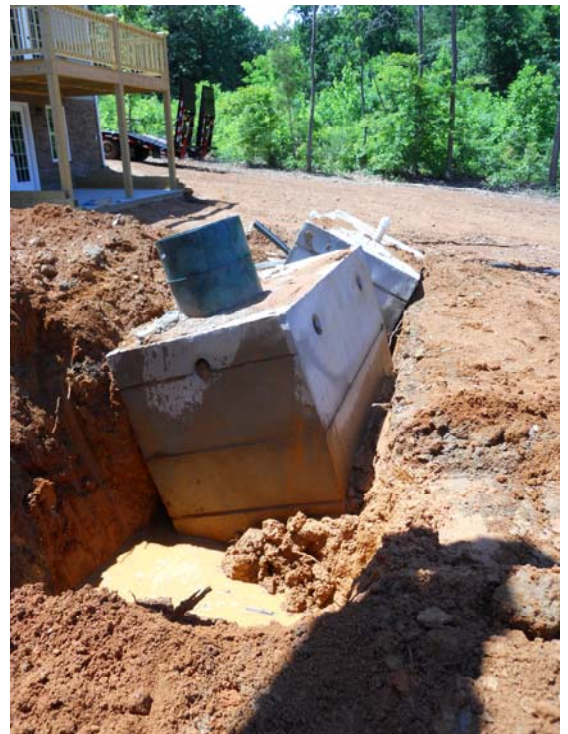
Figure: 7-36. Floating pump chamber. (Photo by Sarah Lewis, EHS)
