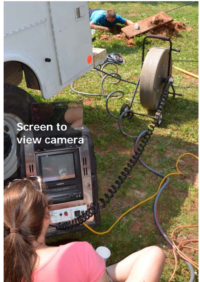
Figure: 7-3. The man in the blue shirt is pushing the camera into the header lines from the distribution box, while the evaluator watches the screen to determine the condition of the system. (Photo by Tom Saxton)
