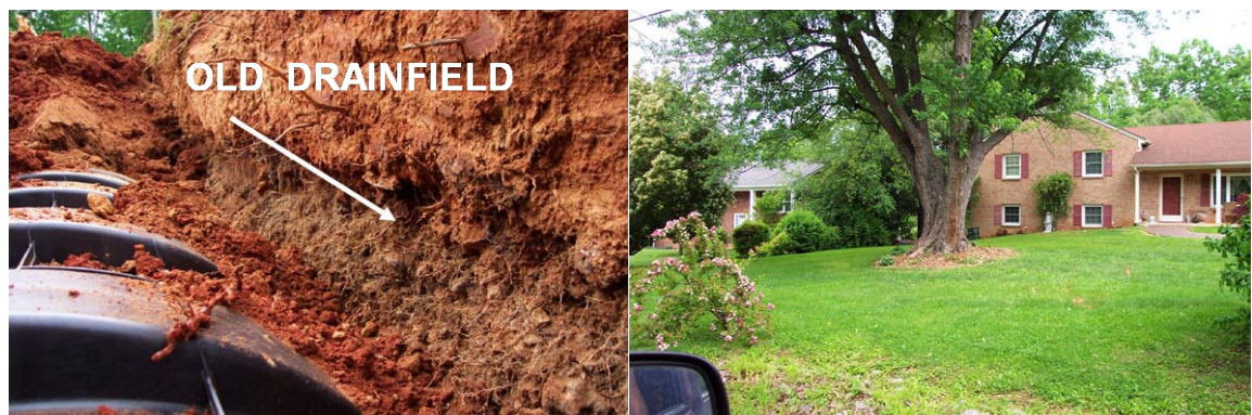
Figure: 6-9B. Root invasion ultimately caused this drainfield to fail. (Photos by Tom Saxton)
