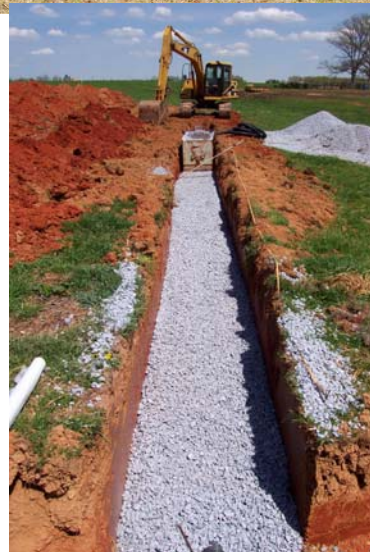
Figure: 7-26. Aggregate trench surfacing patterns. (Photos by Tom Saxton & Gary Gilliam)
