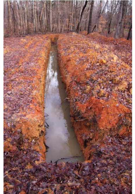
Figure: 6-8. Ponding in trench due to mounding in Mecklenburg County. (Photo by Tom Saxton)
