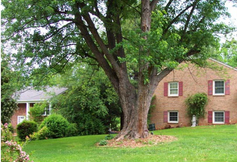
Figure: 7-13. This large maple was planted in the middle of the drainfield. Eventually, the drainfield ceased to function. The upper portion of the drainfield is also higher than the floor level of the lowest plumbing fixture on the lower floor. This caused back ups during heavy precipitation events. (Photo by Tom Saxton)
