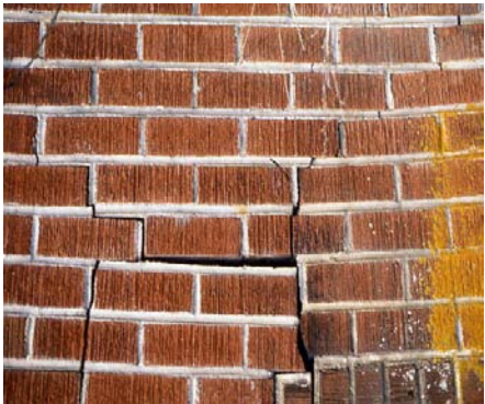
Figure: 5-31. Shrink Swell soils exert tremendous force against foundations. (Photo by Tom Saxton)
