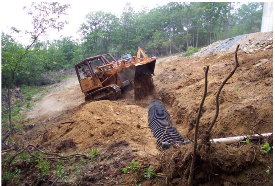
Figure: 7-14. This chamber system could be easily damaged during filling and grading. (Photo by Tom Saxton)
