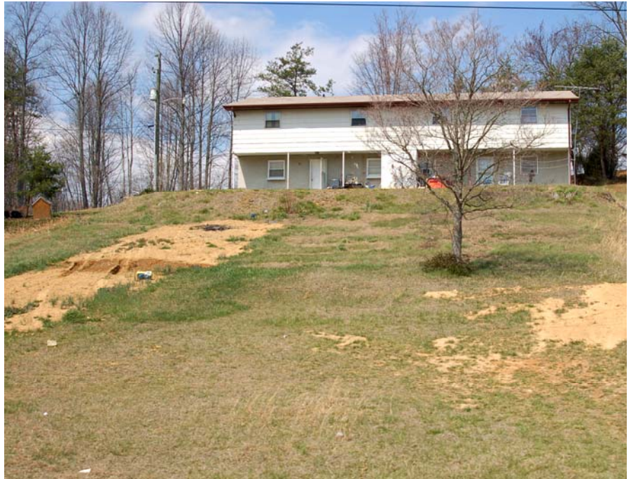
Figure: 7-37. Another common solution is to cover the failed area with soil. As you can see from this photo, that is doomed to failure. The effluent is just wicked up into the fill material. (Photo by Gary Gillian)
