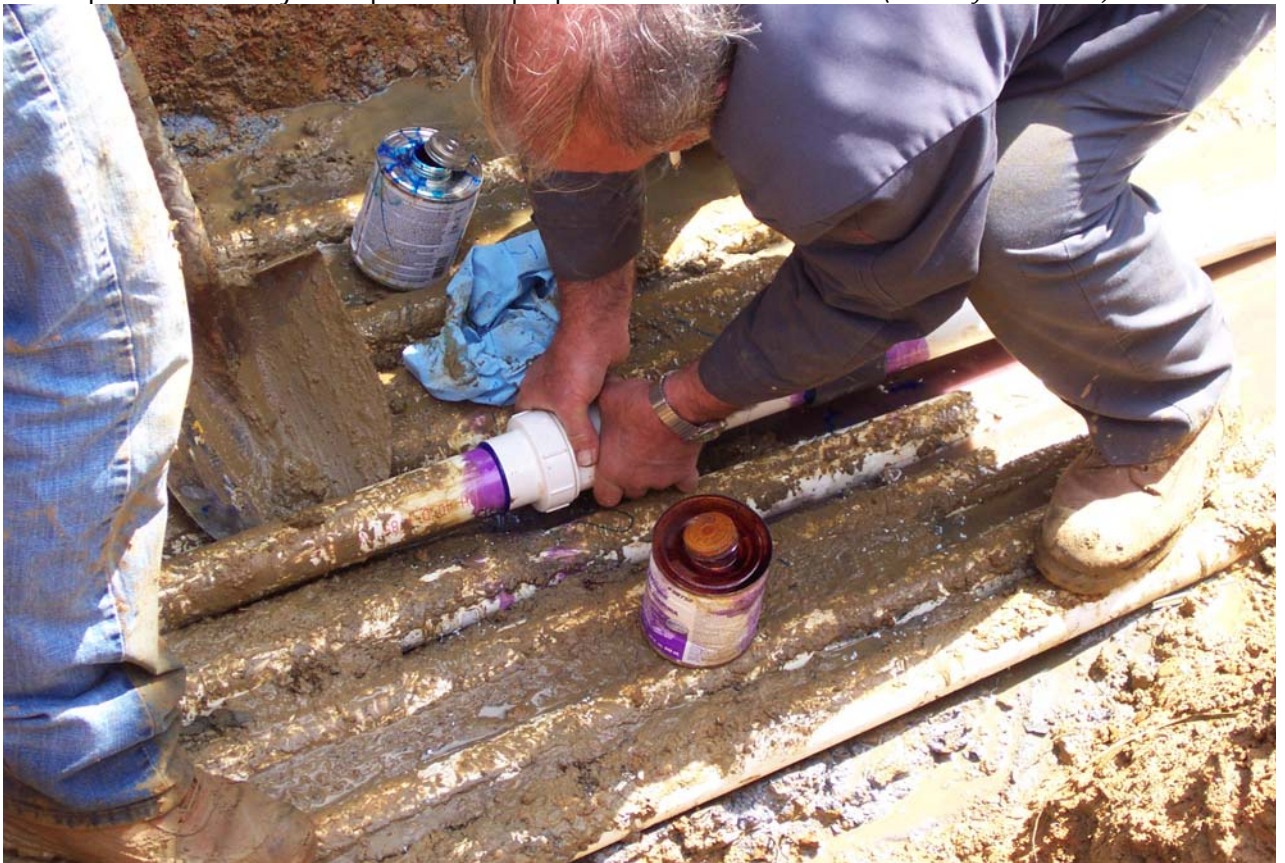
Figure: 7-24. This force main, one of 11, was found to have a linear crack. The difficulty in this case was that all 11 were installed in an easement leading to offsite drainfields. Therefore, 11 homes owned the easement. Who was responsible? Sewage was flowing on the ground. But there was no one to hold responsible in order to repair the failed force main. Ultimately, the original contractors volunteered at their own expense. Offsite systems present unique problems for the evaluator. (Photos by Tom Saxton)
