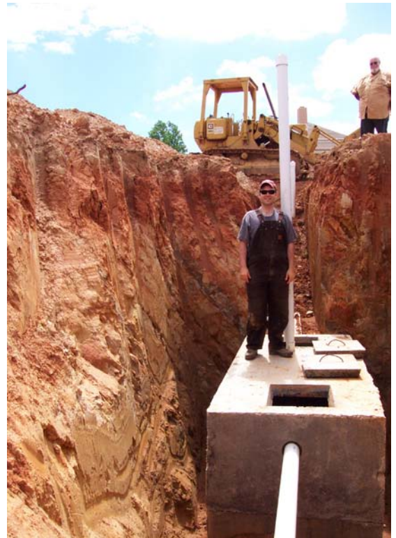
Figure: 6-37. Deep excavations may cave in especially from the vibrations of machinery. (Erik Severson)
