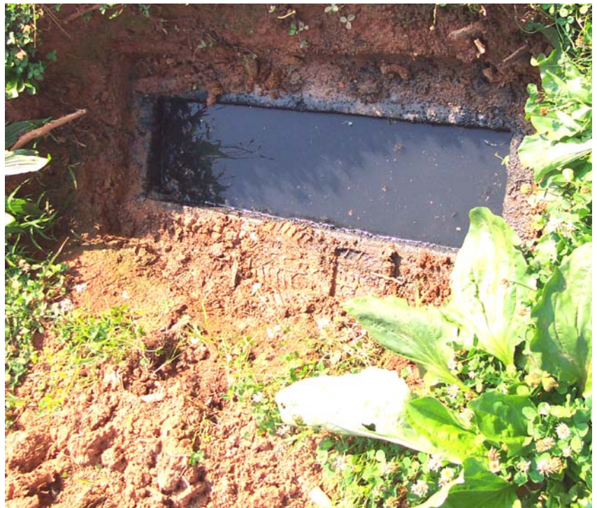
Figure: 7-12. A flooded distribution box indicates that something beyond the box has failed. This could be crushed or root-invaded headers or hydraulically overloaded trenches. (Photo by Tom Saxton)
