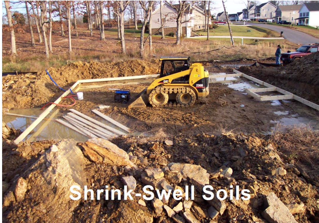
Figure: 6-15. Not only are shrink-swell unsuitable for onsite wastewater systems, they have severe limitations for other uses as well. (Photo by Tom Saxton)
