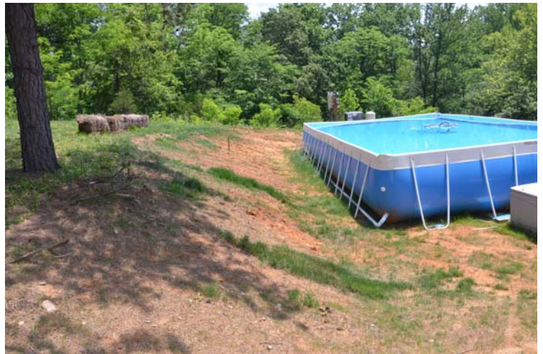
Figure: 7-17. Construction of swimming pools commonly damages a system. In this case, the trench is at the top of the cut bank. Effluent is erupting from the slope. (Photo by Gary Gilliam, EH Supervisor)
