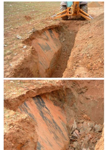
Figure: 5-25. Excavating safety standards must be observed when utilizing test pits for sampling points. Pits may cave in; great caution must be employed during pit evaluations. (Photo by C. M. Allison, Jr., OSE)
