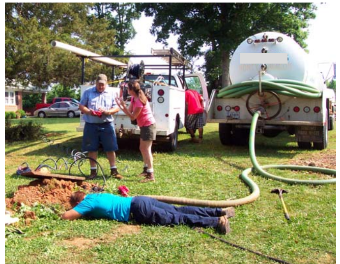
Figure: 7-29. Jetting the lines may help remove solids from pipes thereby extending the life of the system. ( Photo by Tom Saxton )
