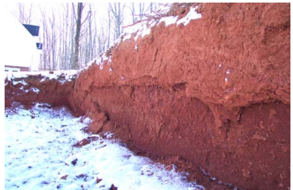
Figure: 6-10. What does the horizontal feature in the middle of this collapsing basement cut imply about soil structure? "Platy" (Photo by Tom
