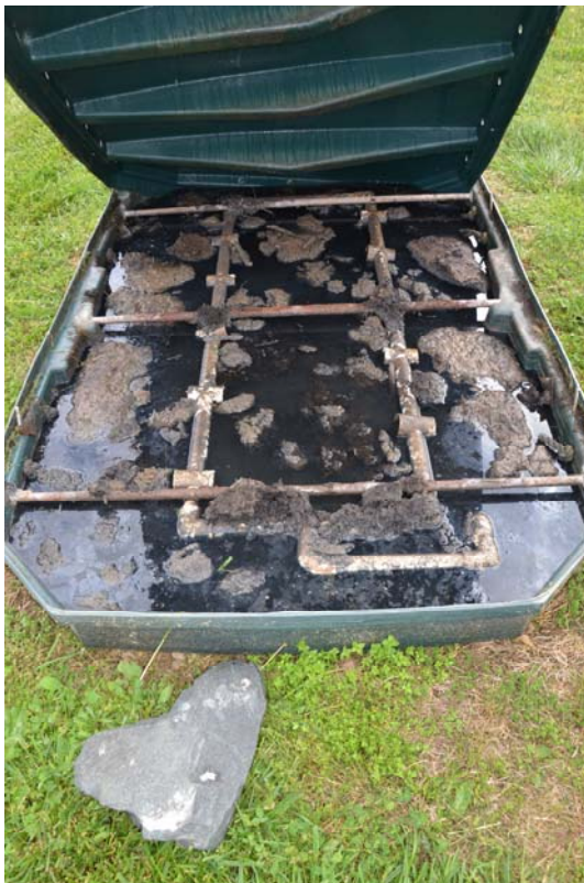
Figure: 7-18. Alternative treatment systems are not immune to problems. In this case, an automotive repair shop's system was compromised by mechanics hand cleaner. (Photo by Tom Saxton)
