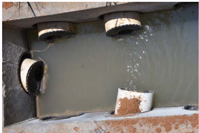
Figure: 7-19. A baffle should be installed to prevent "short-circuiting" preferential flow to one trench. A 90-degree elbow on the inlet may solve this problem. (Photo by Tom Saxton)
