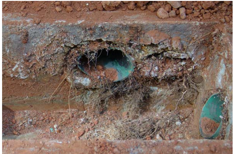
Figure: 7-16. Dissolved distribution box. (Photo by Tom Saxton)
