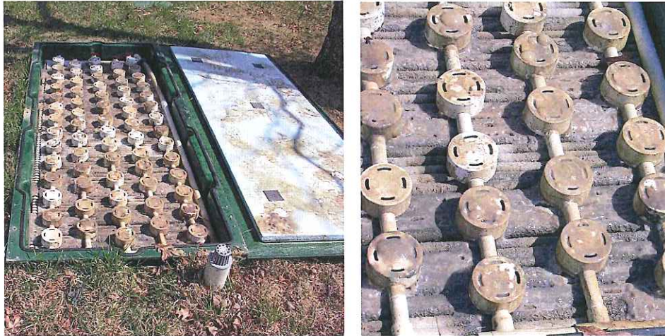
Photograph 5: AdvanTex ® System Receiving Residential Effluent with Water Softener Backwash Brine
