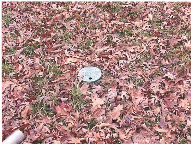
Photograph 4: Completed Lysimeter Installation with Sampling Tubes Enclosed in Valve Box
