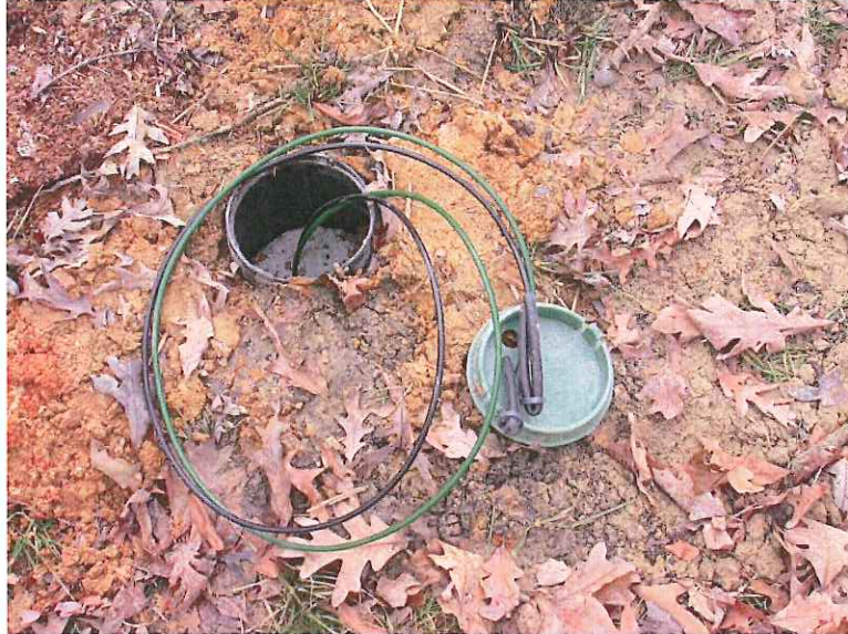
Photograph 3: Completed Lysimeter Installation with Sampling Tubes Exposed
