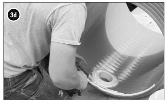
Apply bead of adhesive under RSV bracket
