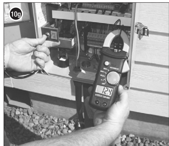
Measure amperage.
