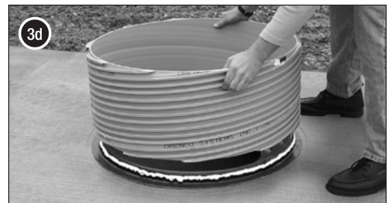
Carefully slide the riser onto the adapter.
