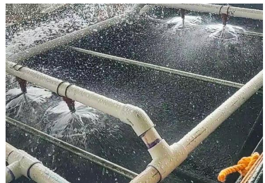
Figure 1: Replacement Grid with Helical Spray Nozzles
