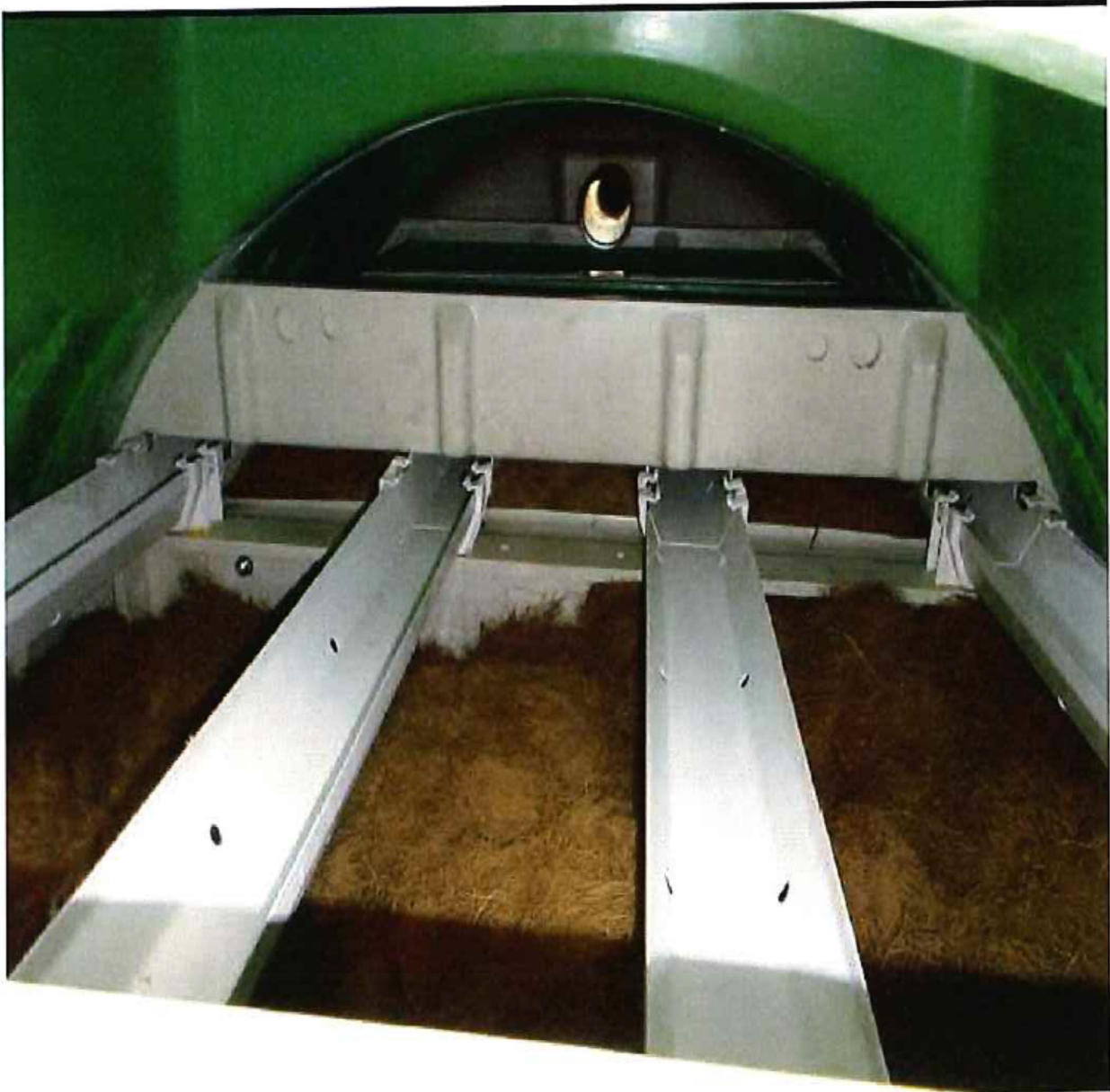
Figure 6: View into the tank with the distribution system and the filter material
