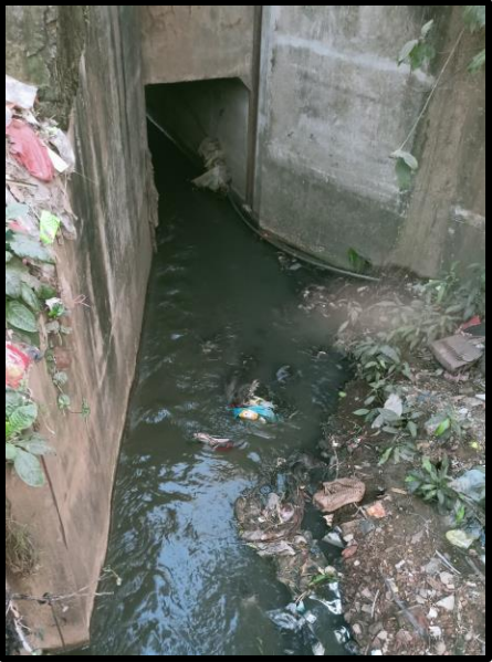
Small Sluice gate
