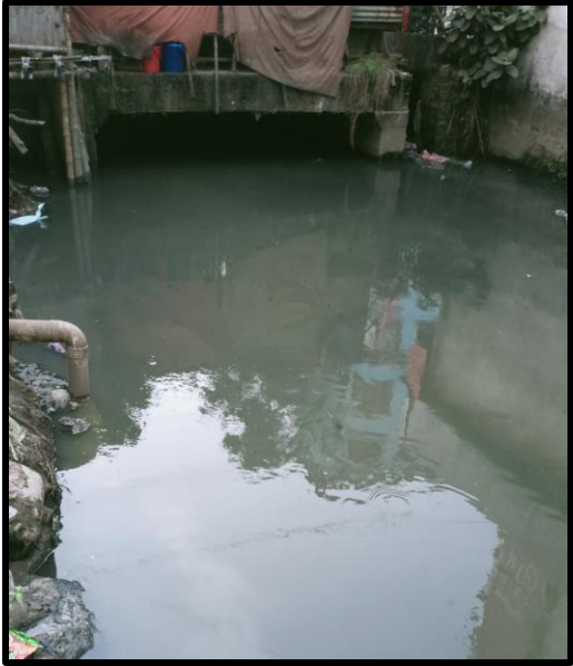
Concrete Open Canal
