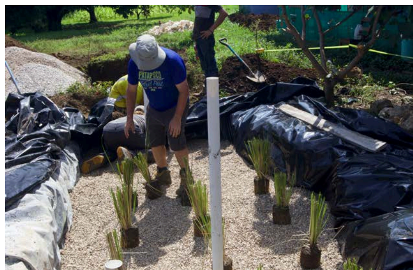
Biochar is mixed throughout the gravel and woodchip layer
