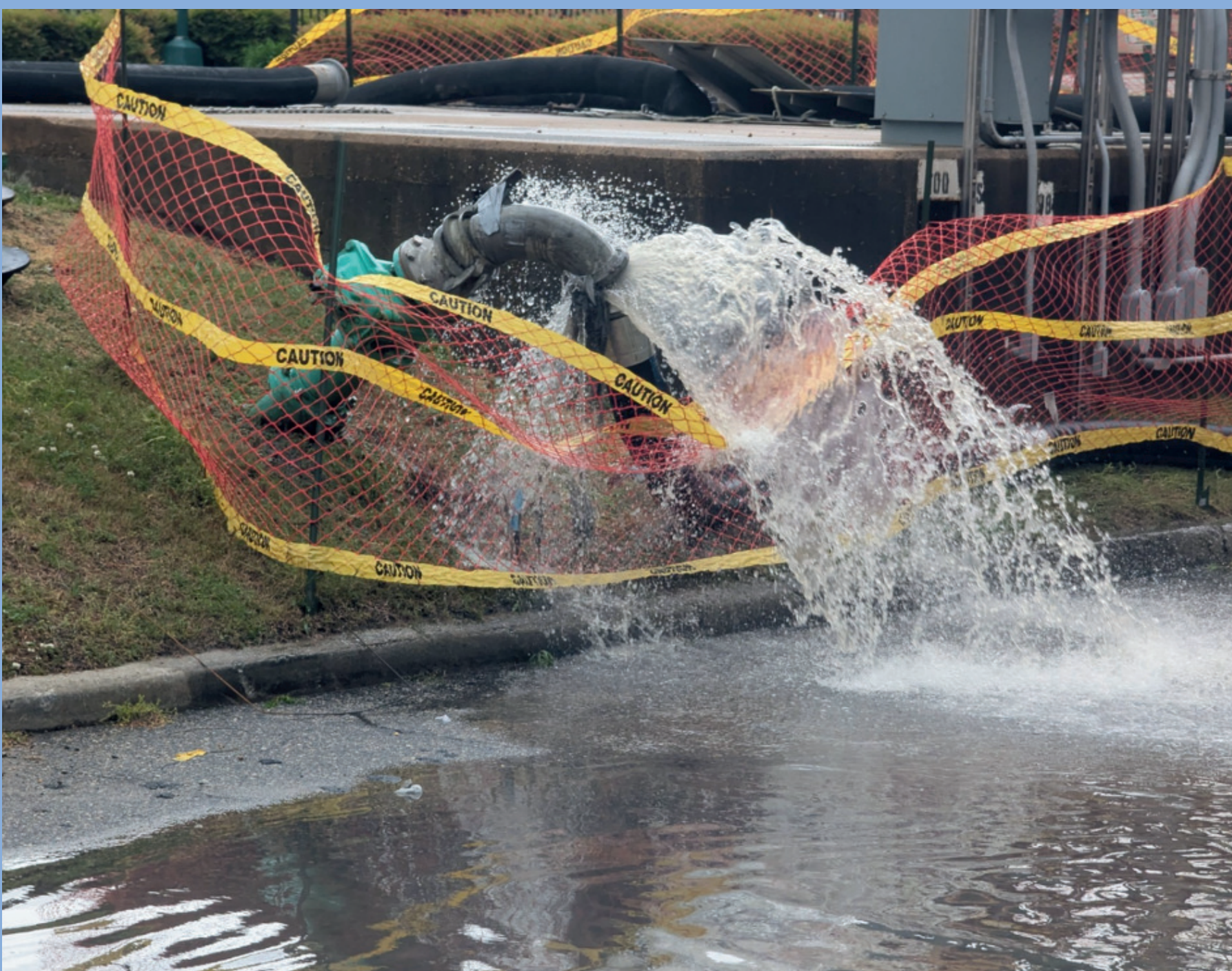
Raw Wastewater Spill in Norfolk
