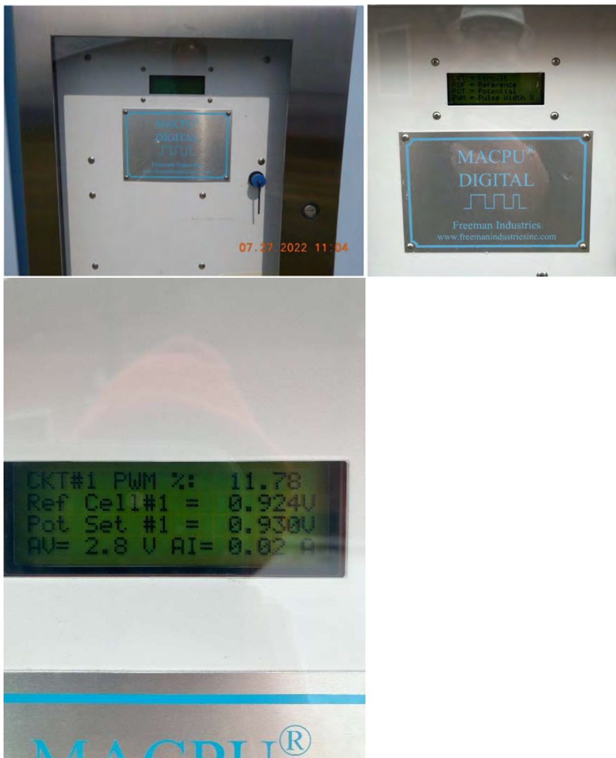
Figure 66. Cathodic Protection Unit at Cofer Road tank (Top left-EPA, Top right- COR, Bottom- VDH)
