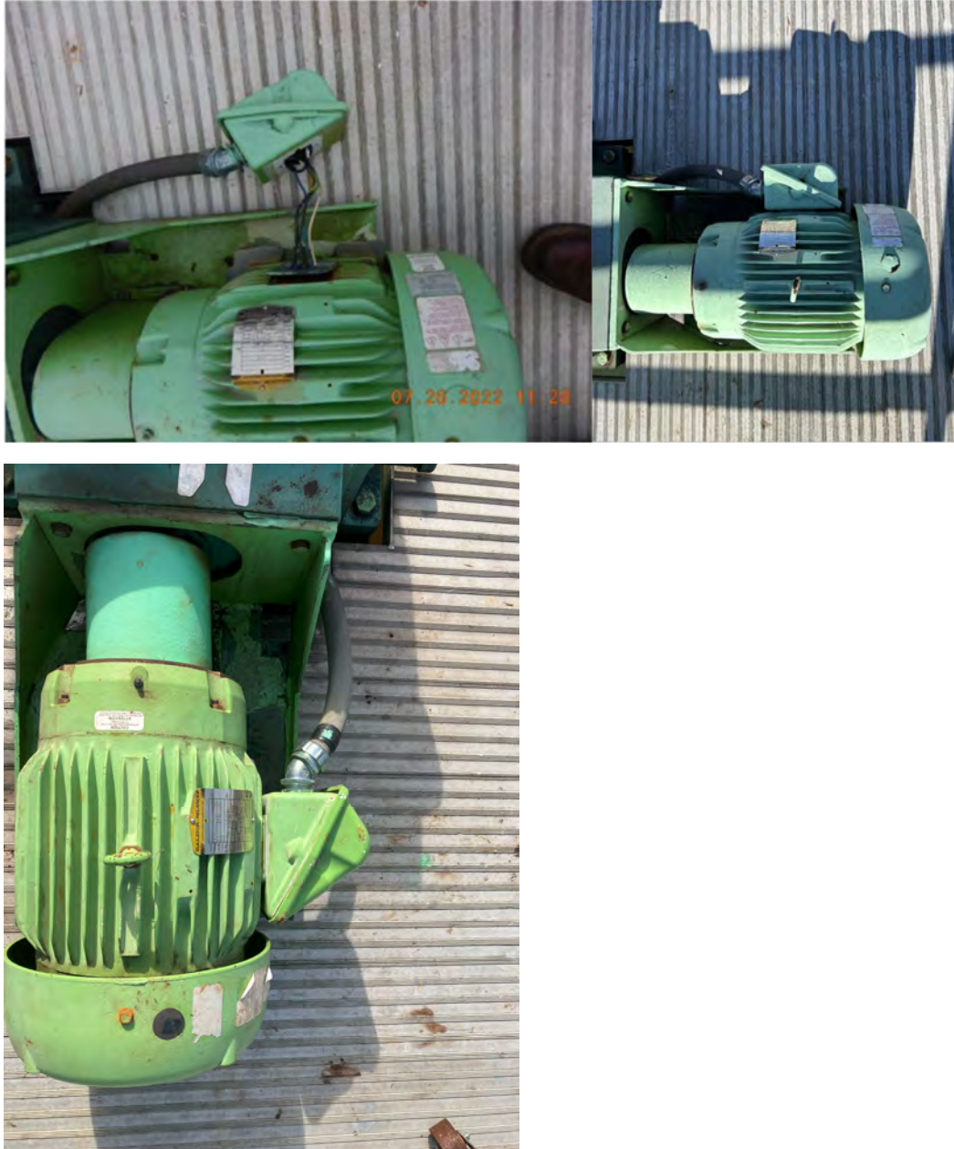
Figure 55. Exposed wiring flocculator motor (Top Left-EPA, Top Right-COR, Bottom Left- VDH)
