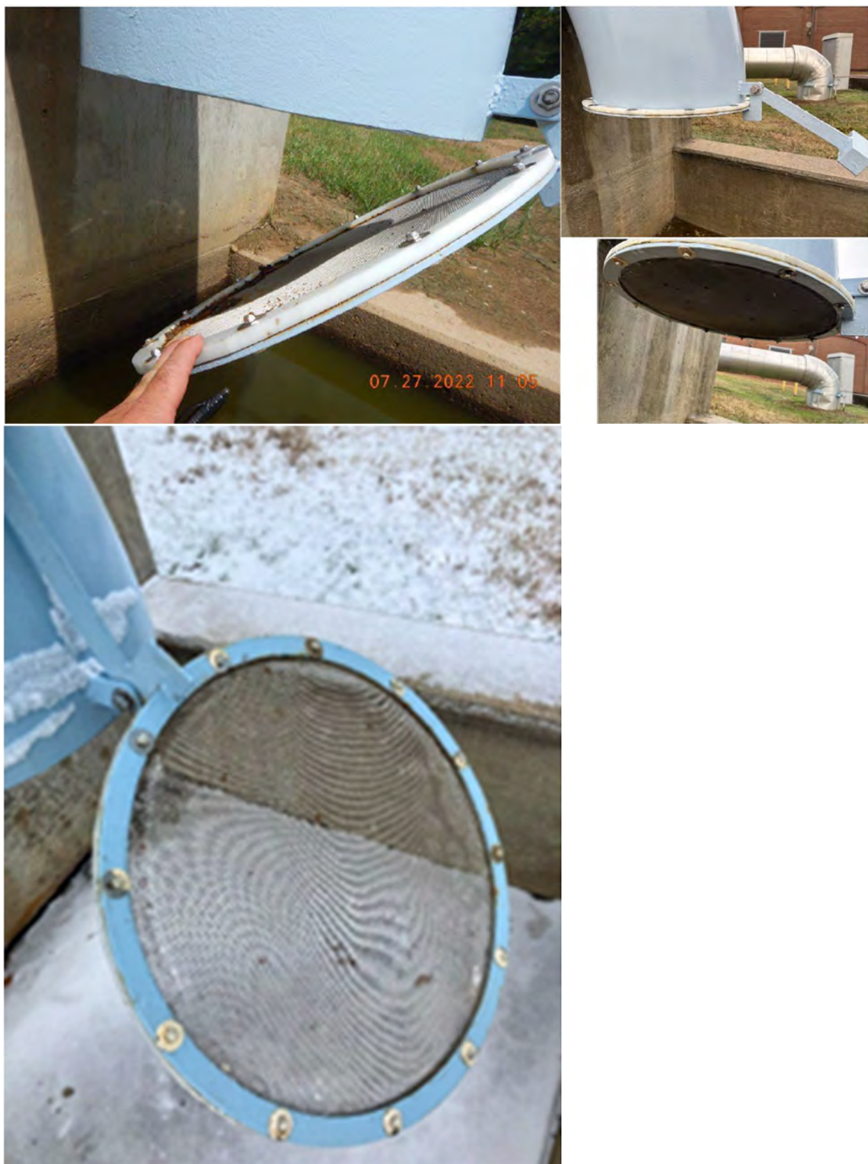
Figure 31. Cofer Road overflow screen (Top left-EPA, Top right-COR, Bottom-VDH, Fine Mesh (also has air gap of ~3 feet))
