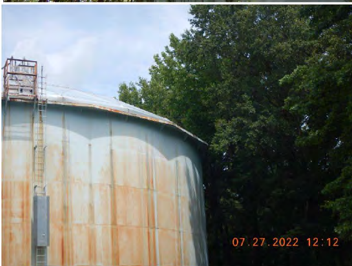
Figure 39. Storage tank vegetation and overgrowth (EPA)
