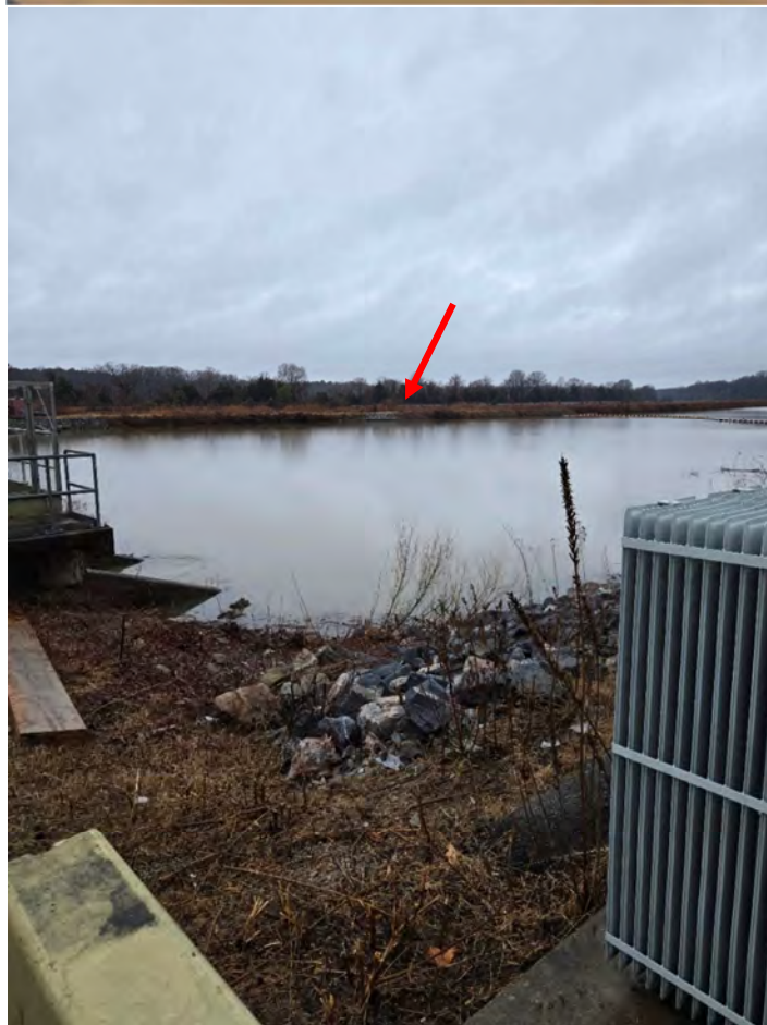
Figure 48. Earthen berm between lagoon and raw water intake channel (VDH)
