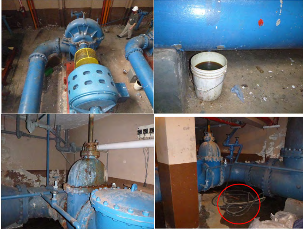
Figure 36. Byrd Park Main Pump Station debris, leaks, housekeeping, backflow prevention (EPA)
