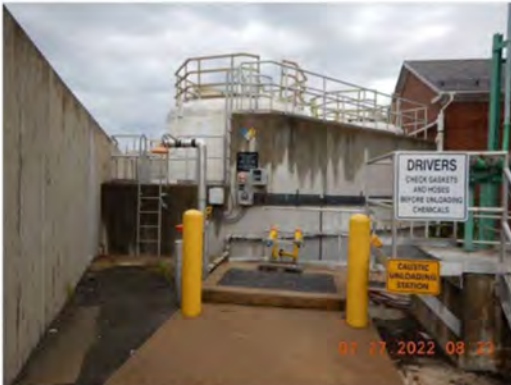
Photograph 37. Caustic soda bulk storage area adjacent to the Korah 1 Pump Station
