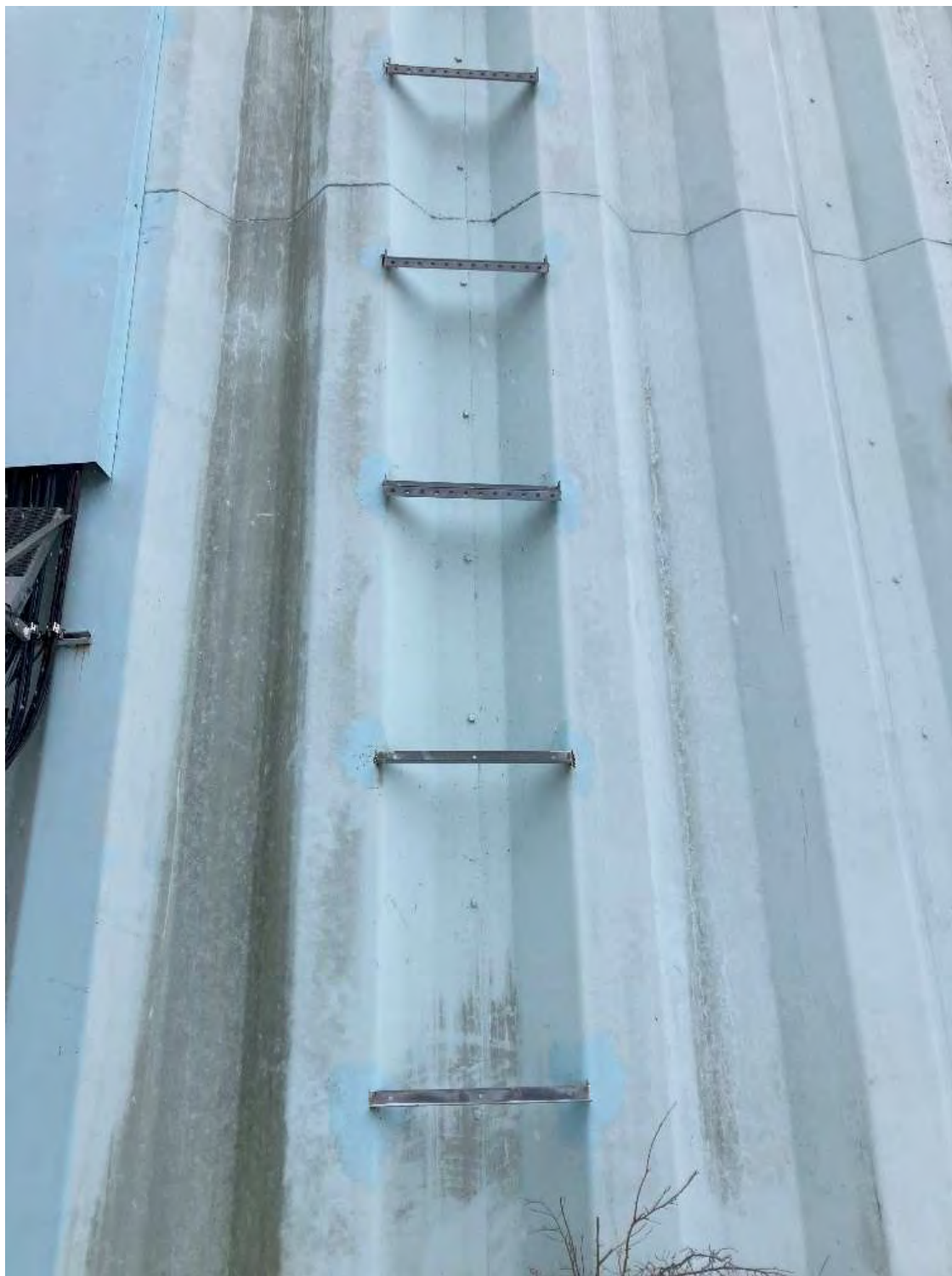
Figure 71. Warwick Tank unprotected access to top of tank (VDH)
