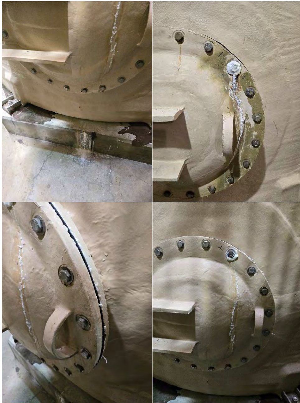
Figure 13. Leaks observed in sodium hypochlorite tanks (VDH)
