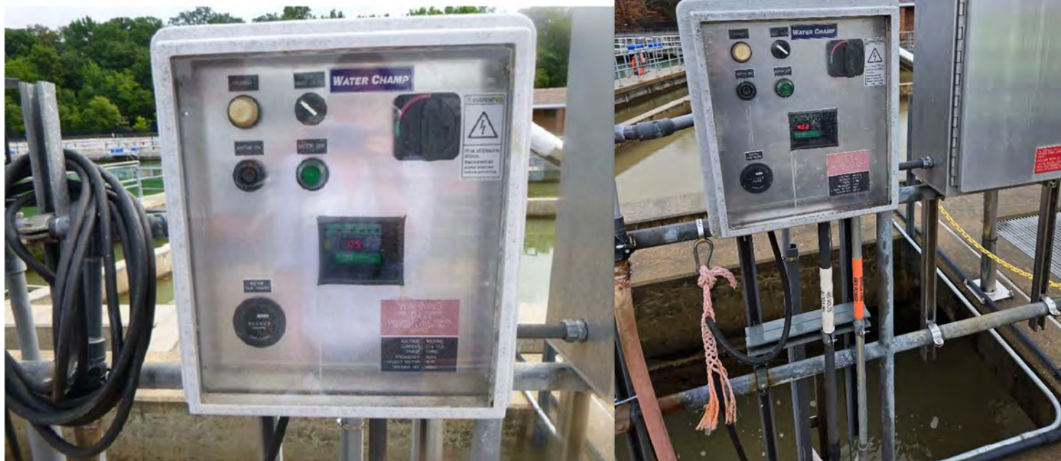
Figure 87. Water Champ flash mixer controls (Left- EPA, Right- VDH)
