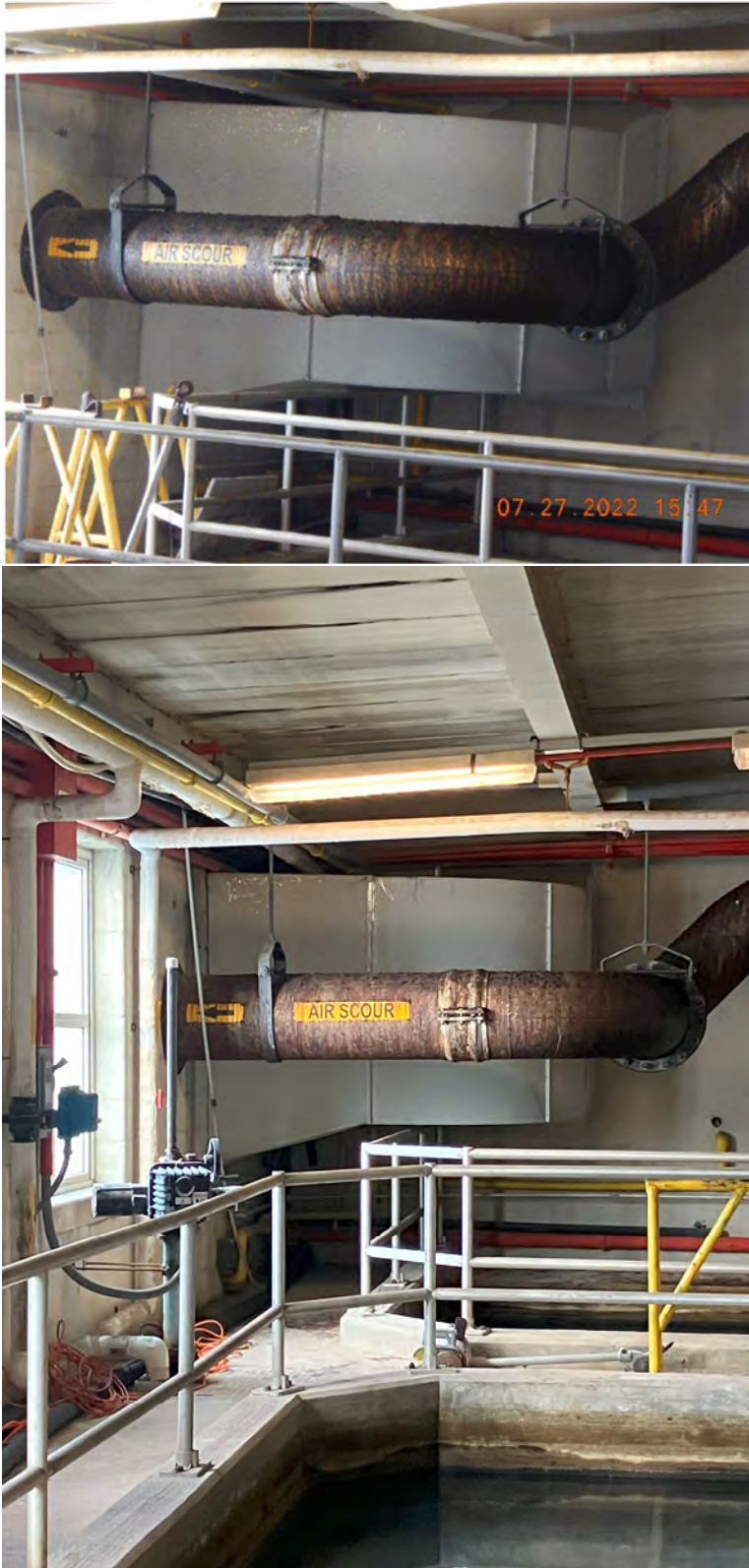
Figure 19. Plant 1 air scour piping (Top- EPA, Bottom-VDH)
