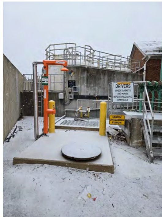
Figure 88. Caustic soda bulk storage area (Top Left- EPA, Bottom Left- COR, Right- VDH)
