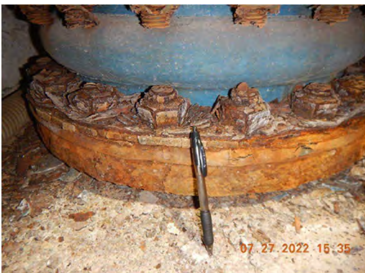
Figure 21. Corrosion at filtered water pumps (EPA)
