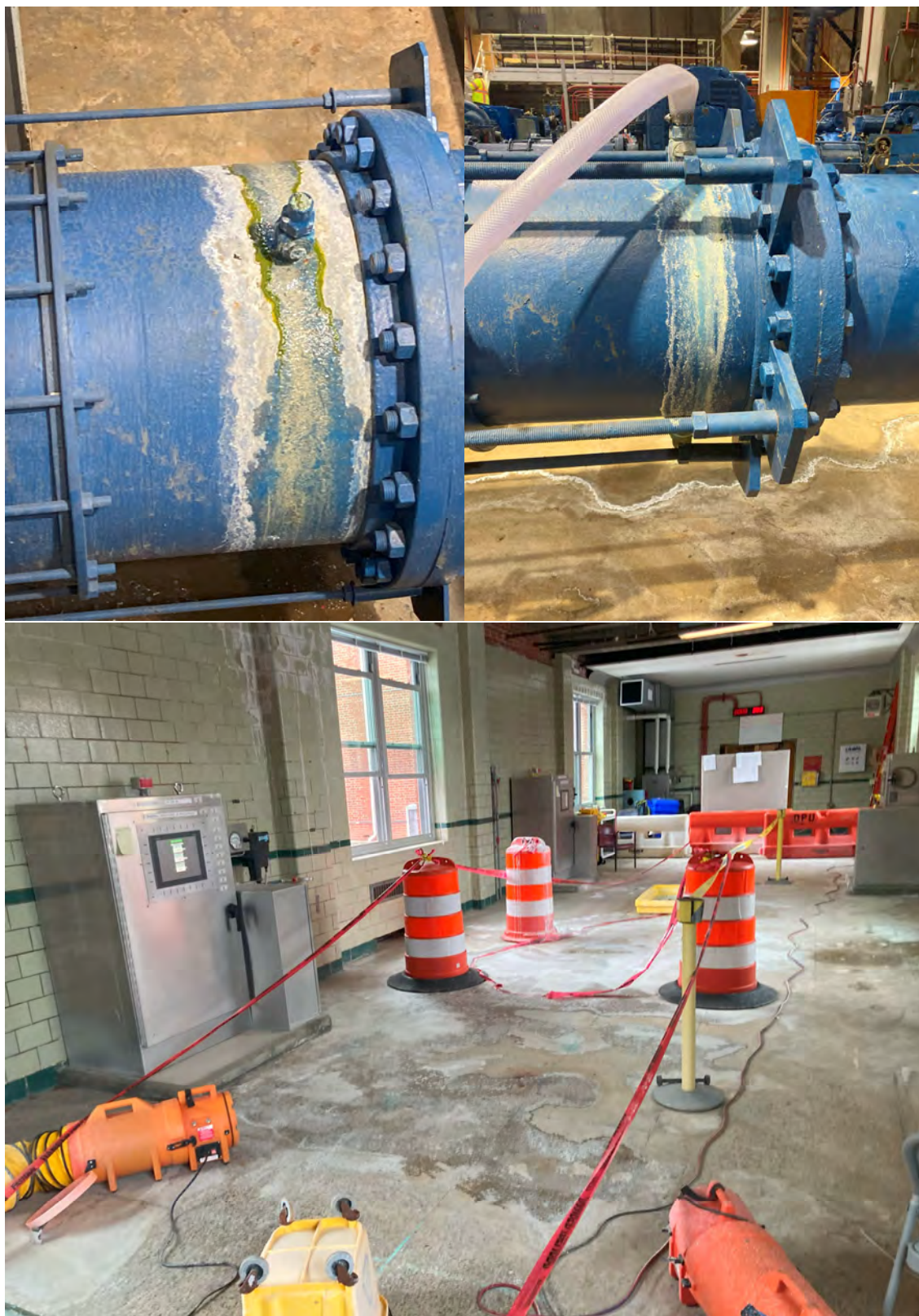
Figure 10. Chemical leaks observed (VDH)
