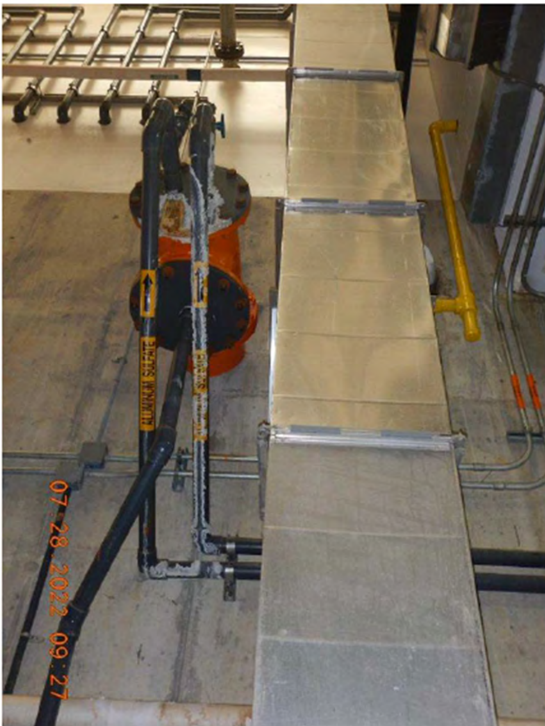
Figure 82. Aluminum sulfate day tank supply line (EPA)
