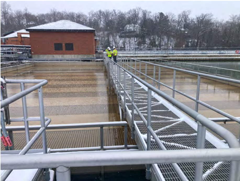
Figure 54. Plate settlers (Top- EPA, Bottom- VDH)
