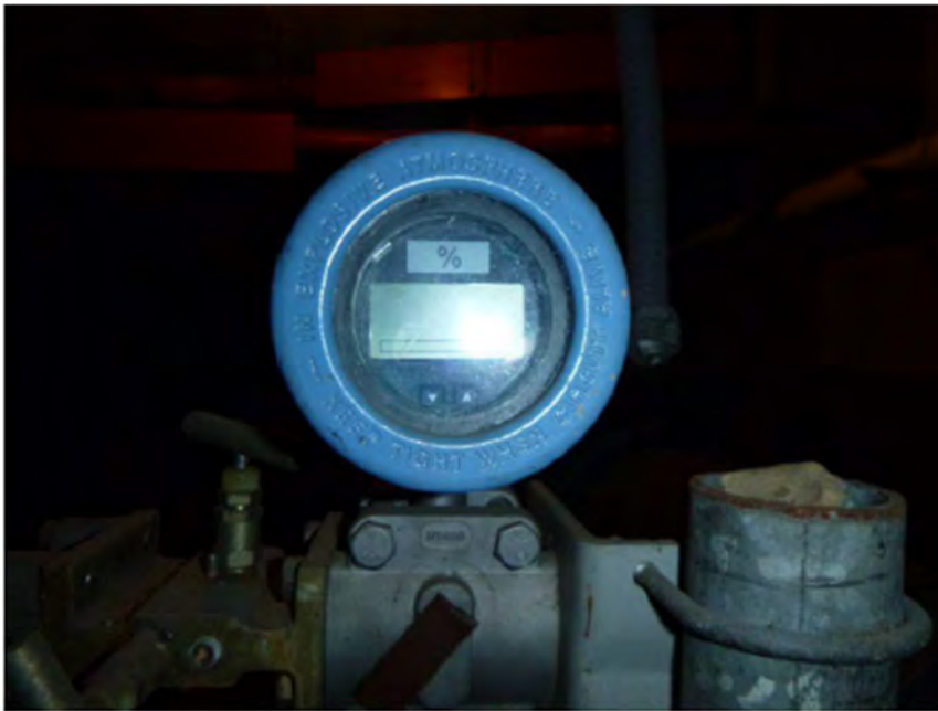
Figure 91. Gauges and flow meters in Byrd Park main pump station not operational (Left-EPA, Middle- COR)
