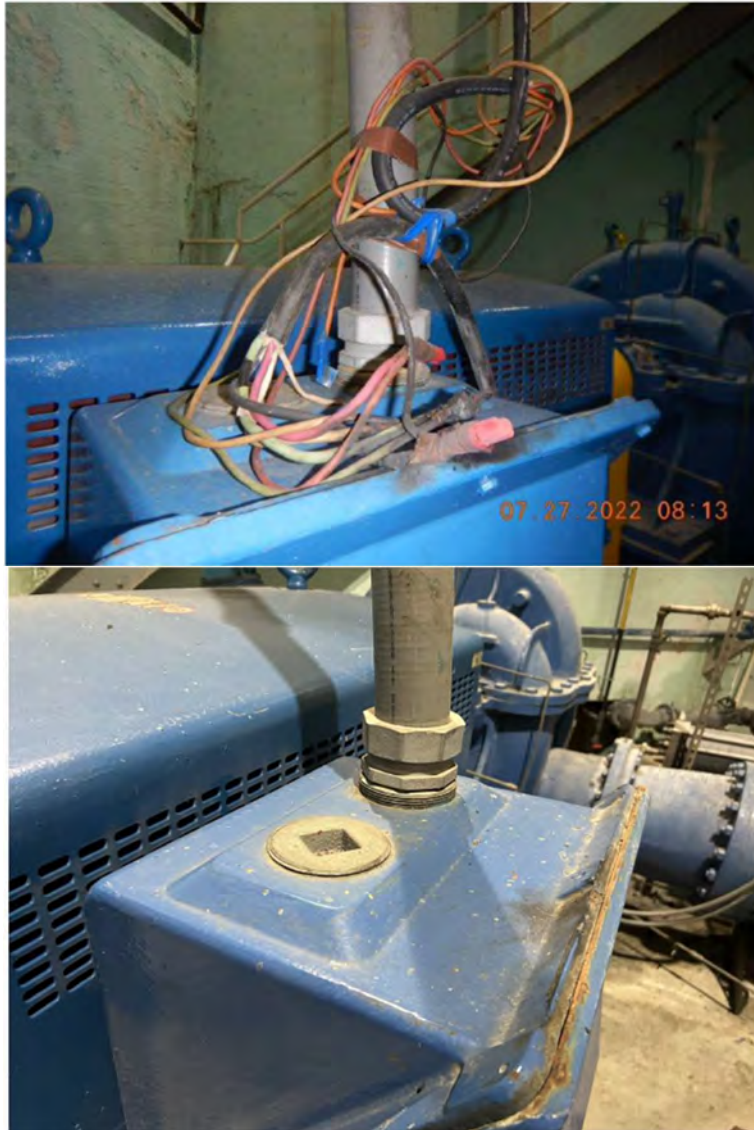
Figure 60. Exposed wiring Korah 1 pump station (Top-EPA, Bottom-COR)
