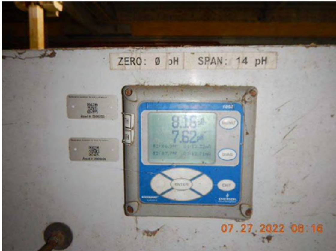
Figure 58. Korah 1 Pump Station pH analyzers (EPA)
