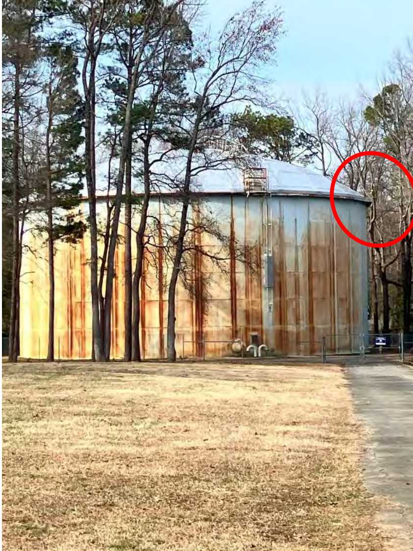
Figure 41. Storage tank vegetation and overgrowth. Cut limbs visible (VDH)
