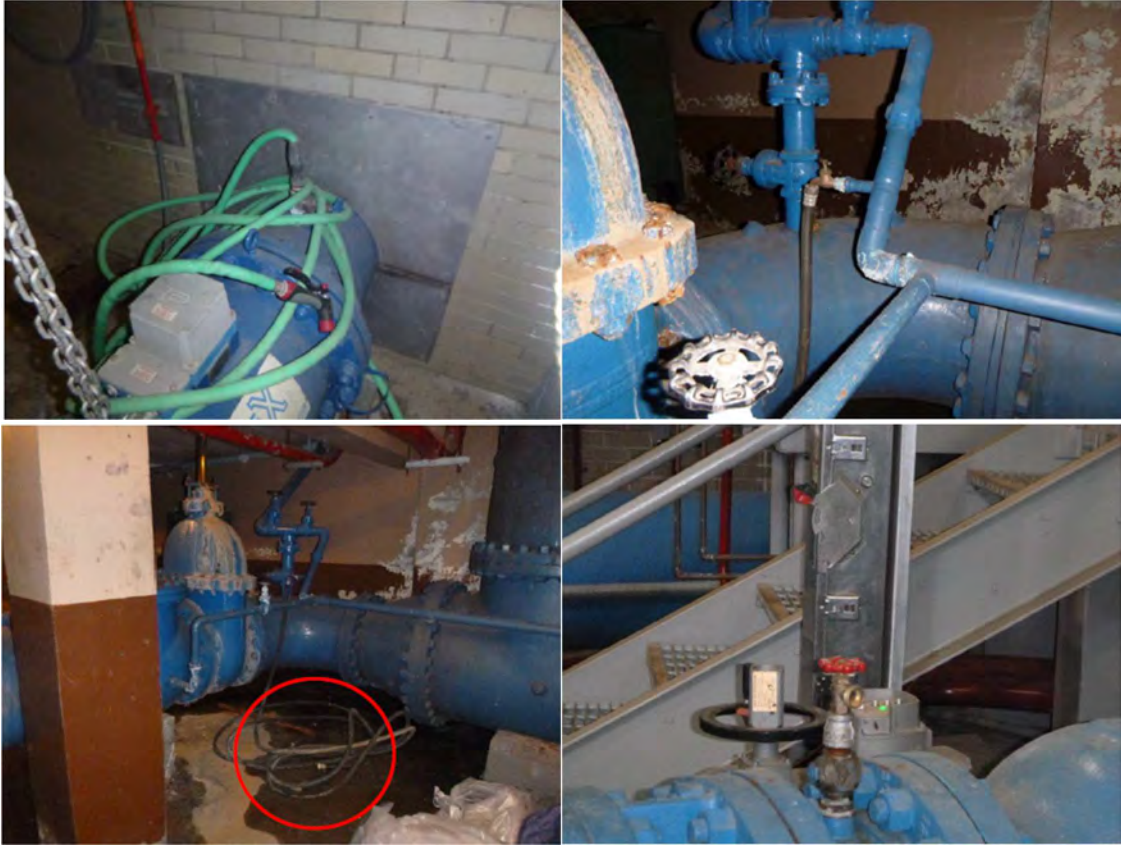
Figure 46. Threaded taps on lines without vacuum breaker (EPA)
