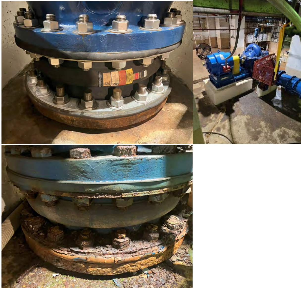
Figure 23. Filtered water pumps mix of upgrades and old corrosion observed (VDH)
