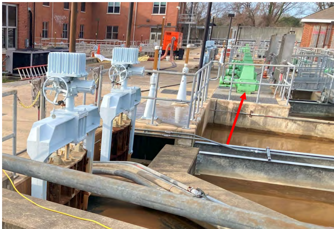
Figure 6. Rapid mix units that can be used as backup for inline mixers (VDH)
