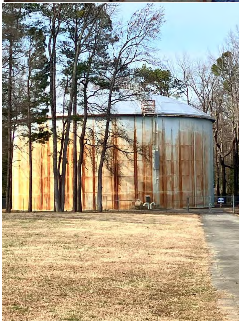
Figure 68. Rust observed on Jahnke Road Tank (Top-EPA, Bottom-VDH)
