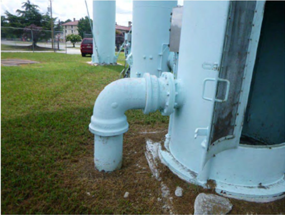
Figure 80. Ginter Park tank overflow pipe (EPA)
