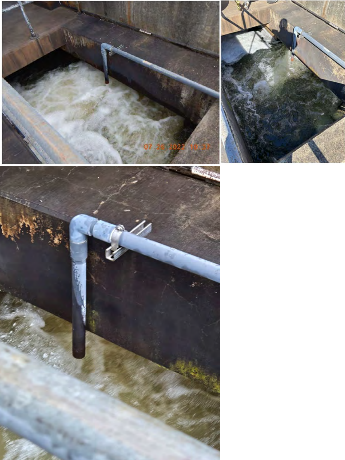
Figure 8. Potassium permanganate feed (Top left- EPA, Top right- COR, Bottom- VDH (not used in winter))
