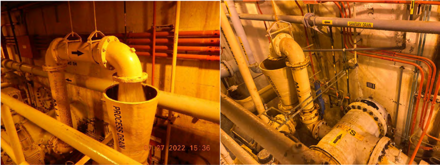
Figure 89. Process Drain (Left-EPA, Right-VDH)
