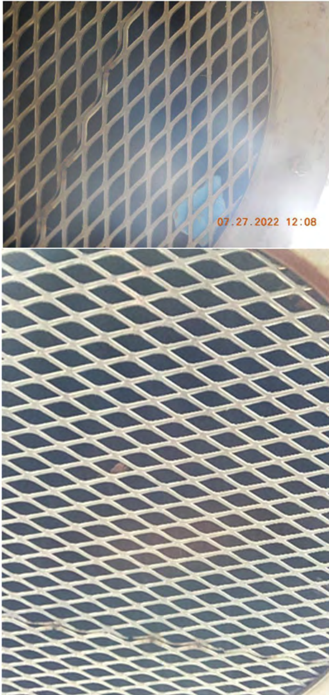
Figure 32. Jahnke Road overflow screen (Top-EPA, Bottom-VDH)
