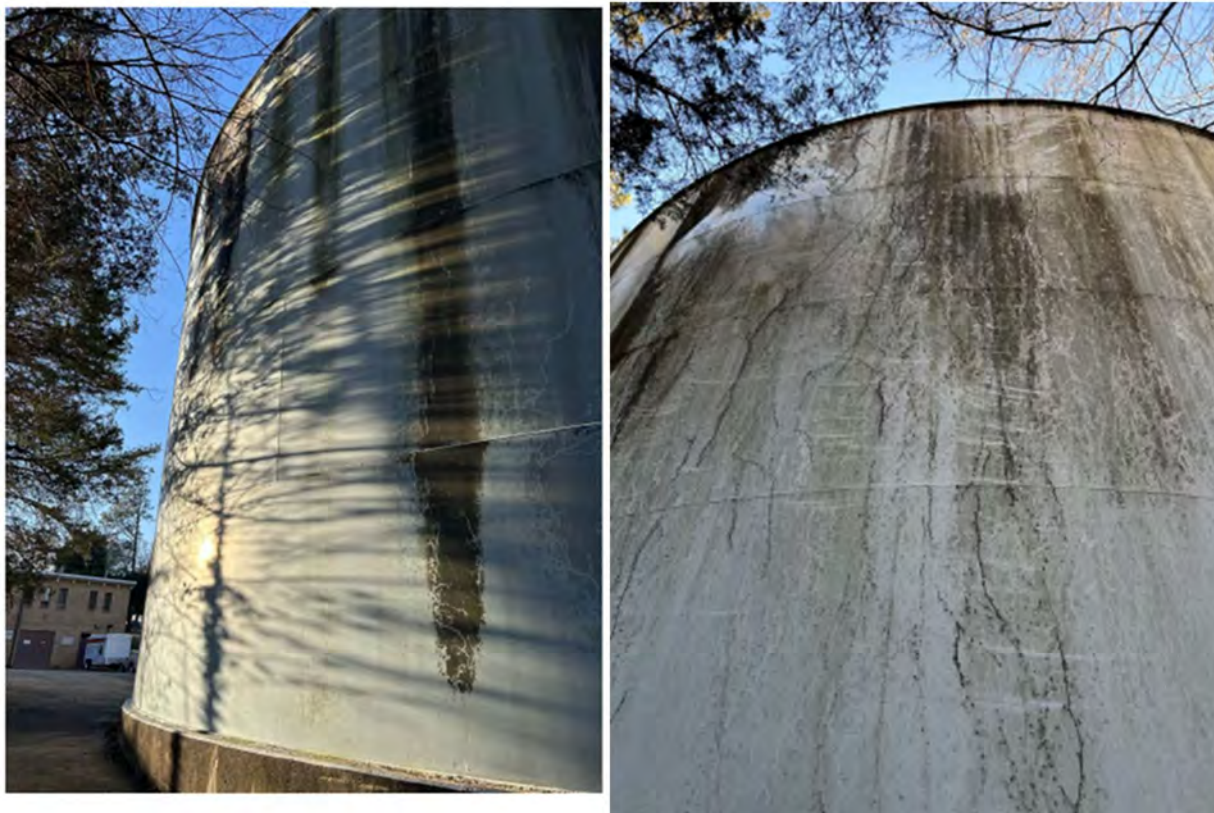
Figure 40. Storage tank vegetation and overgrowth (COR)
