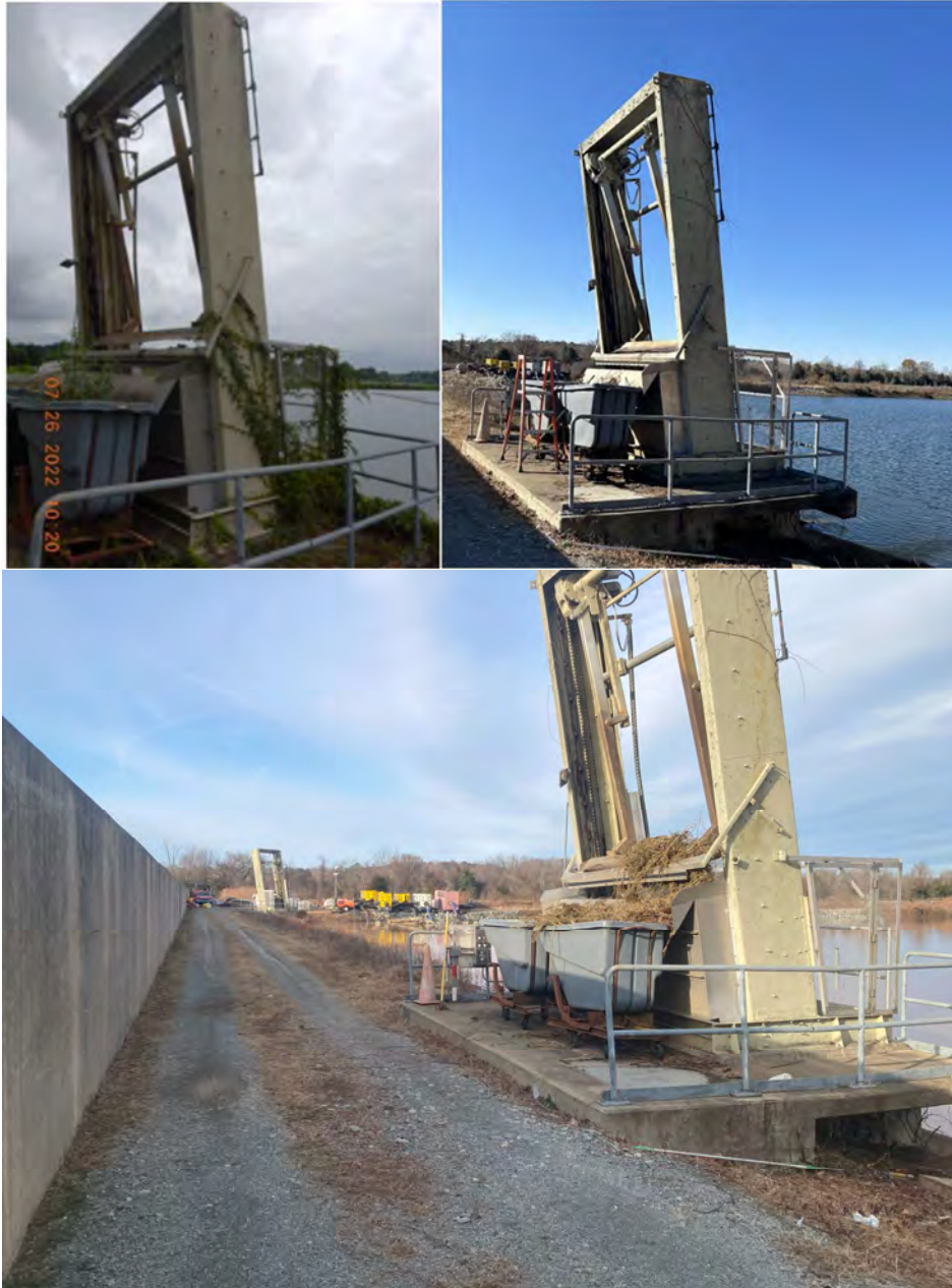
Figure 49. Raw water screens (Left-EPA, Middle- COR, Bottom-VDH)
