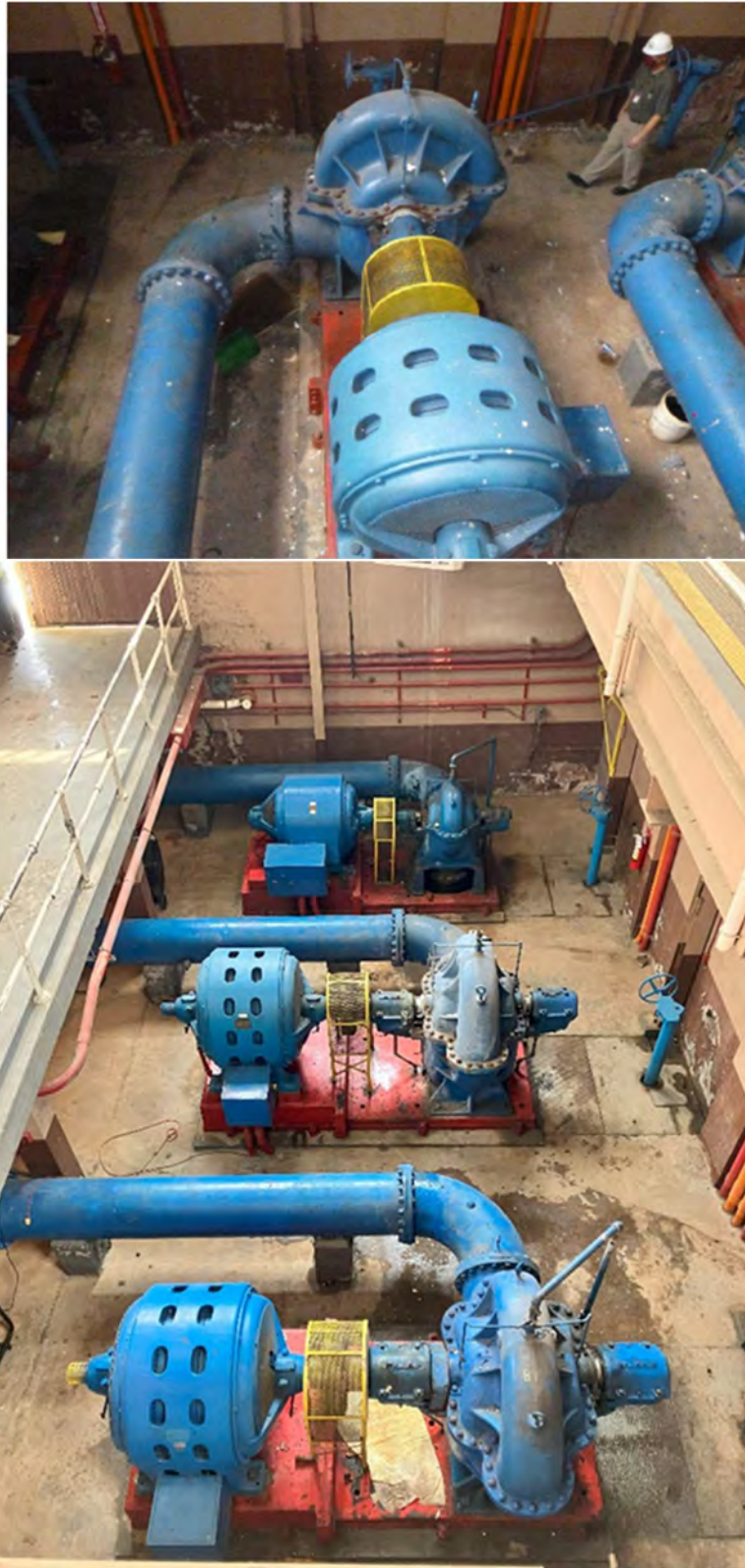
Figure 77. Debris on ground from ceiling at Byrd Park Main pump station (Top- EPA, Bottom- VDH)
