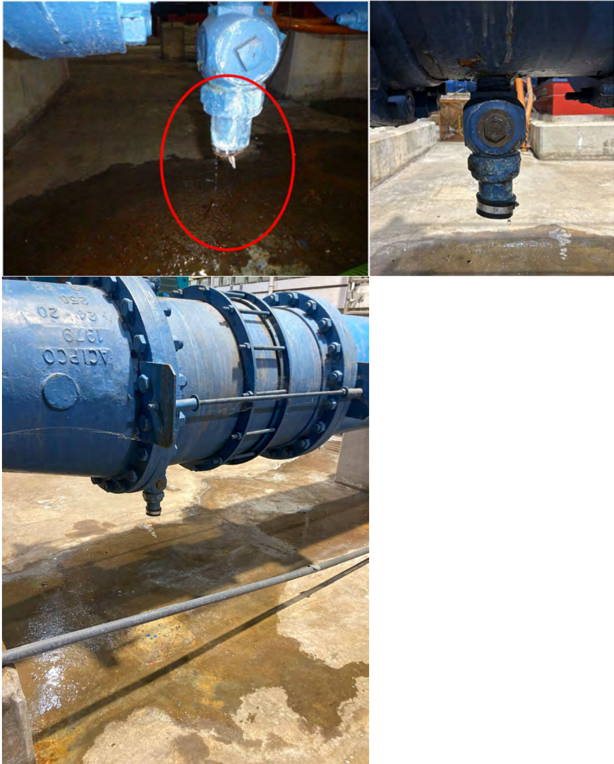
Figure 62. Corroded fitting from pipe in Korah 2 and 3 pump station (Top left- EPA, Top right- COR, Bottom- VDH)
