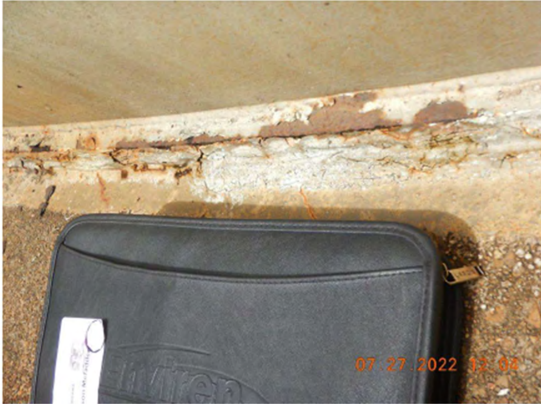
Figure 69. Corrosion and degraded seal at Jahnke Road Tank (EPA)
