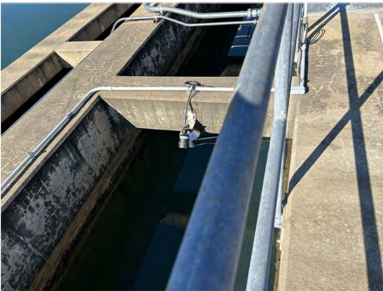
Figure 7. Plant 2 flow meter (Top- EPA, Bottom- COR)
