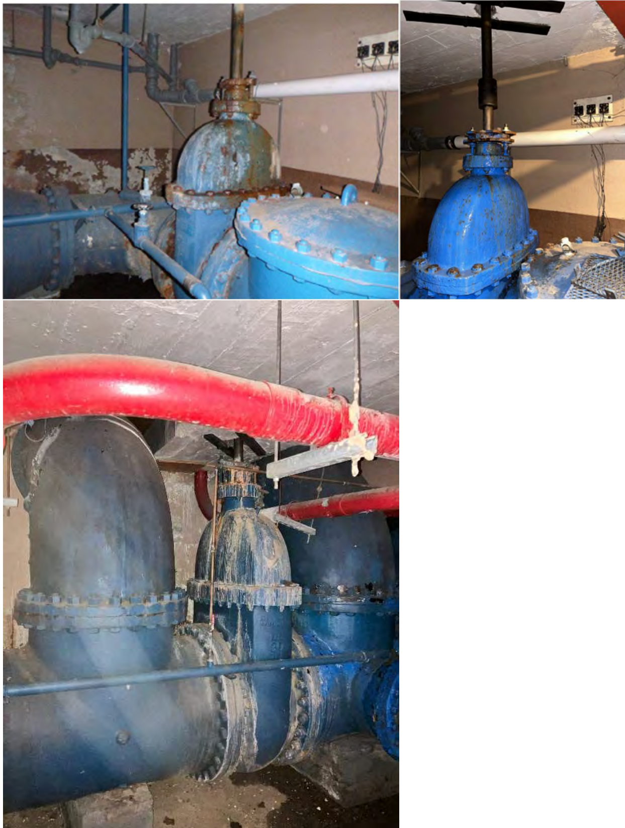
Figure 78. Leaking seals on gate valves at Byrd Park Main pump station (Top left- EPA, Top right- COR, Bottom- VDH)
