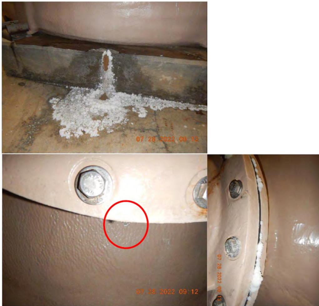
Figure 11. Leaks observed in sodium hypochlorite tanks (EPA)
