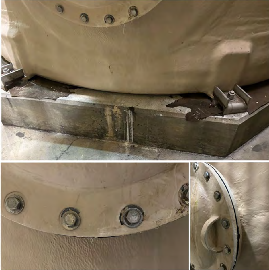
Figure 12. Leaks in sodium hypochlorite tanks (COR)
