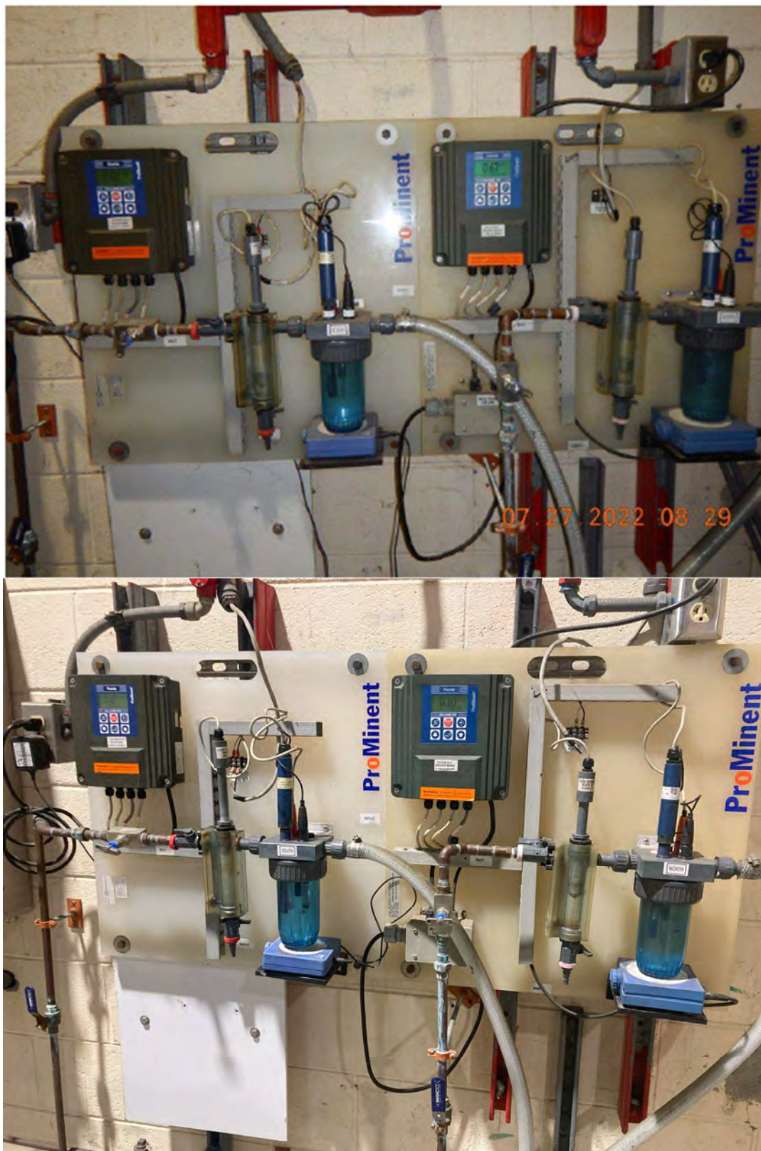
Figure 61. Instrumentation in Korah 2 and 3 pump station, no calibration stickers observed (Top-EPA, Bottom-VDH)
