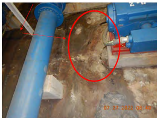
Photograph 44. Water flowing across floor near K3-2 pump, and algal growth on floor near pump motor in Korah 2 and 3 Pump Station.
