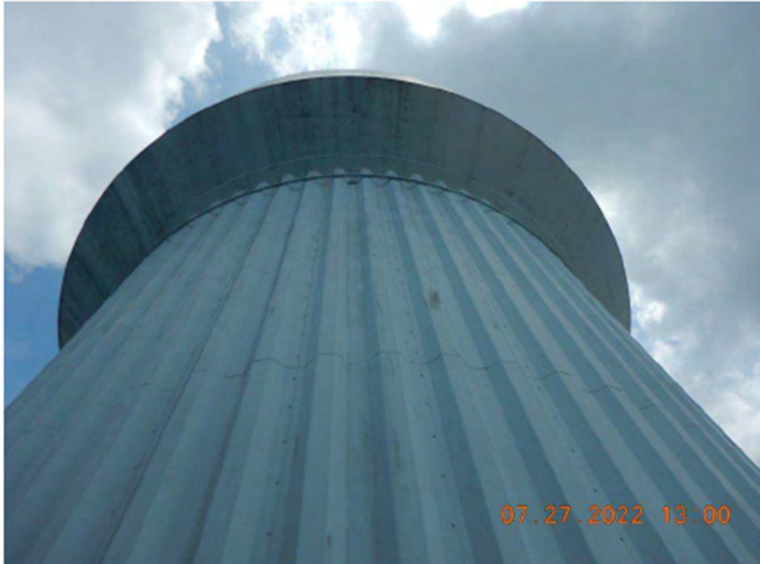
Figure 70. Algal growth at bottom of bowl Warwick Road Tank (EPA)
