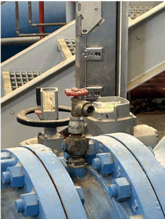
Figure 47. Threaded taps on lines with vacuum breaker installed (COR)
