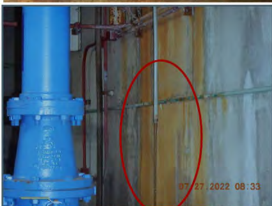
Photograph 43. Process water pipe discharging water on lower level of Korah 2 and 3 Pump Station
