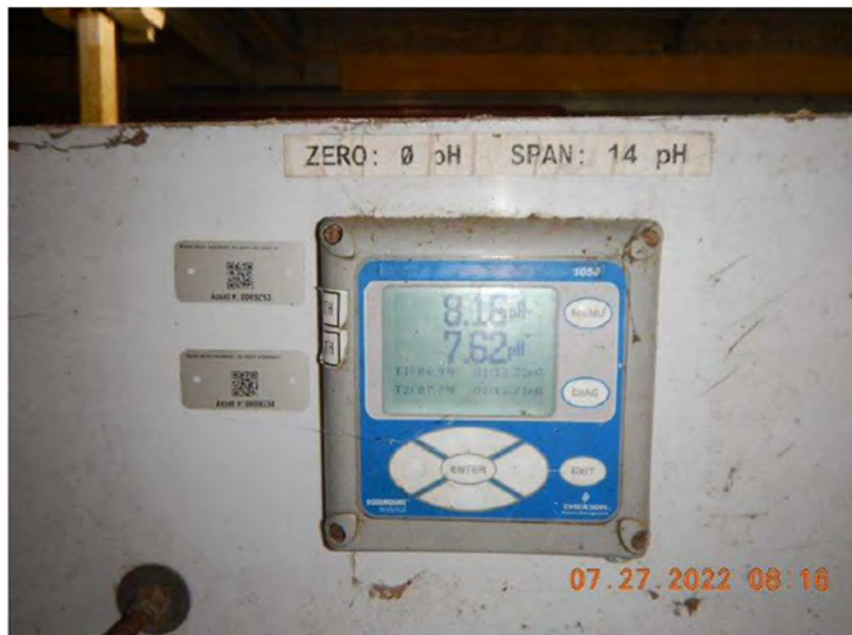
Figure 90. Korah 1 Pump Station pH analyzers (Left- EPA, Right- VDH)
