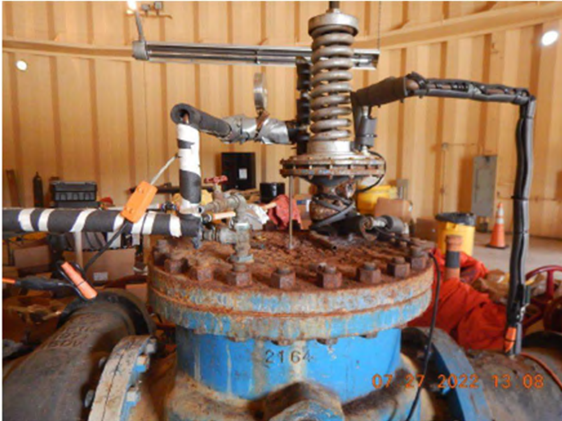
Figure 72. Corrosion on control valve in Warwick Road Tank (EPA)
