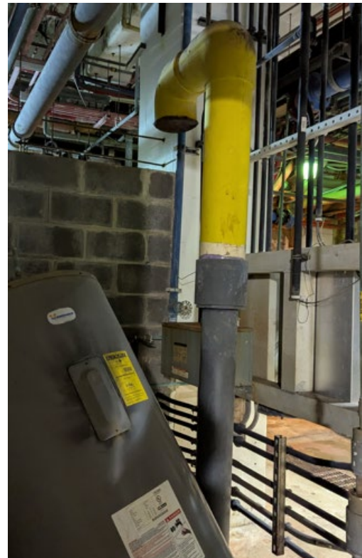
Vent Pipe in Plant #1
