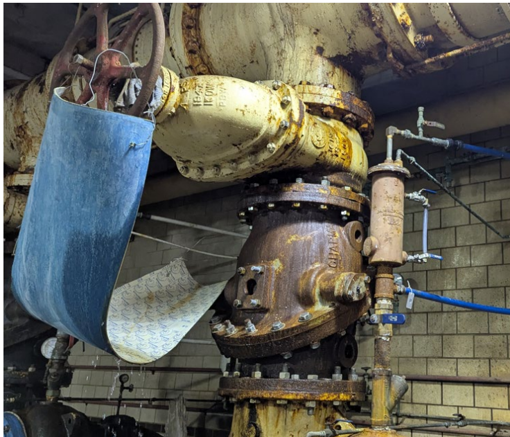
Leaking Gate Valve with Diverter
