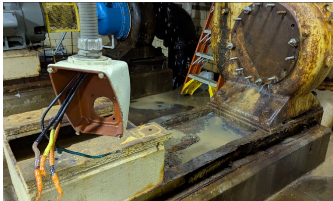
Wastewater Pump No. 2 Motor Missing
