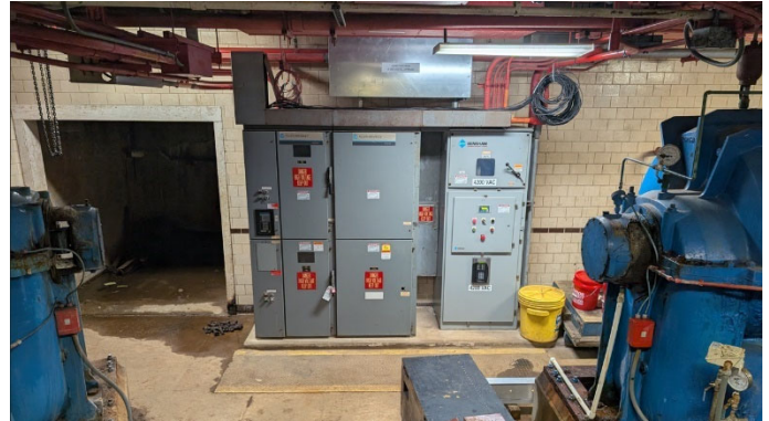
4160V MCC and Variable Frequency Drive – South Filter Plant
