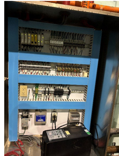
Pump Control Panel Interiors
