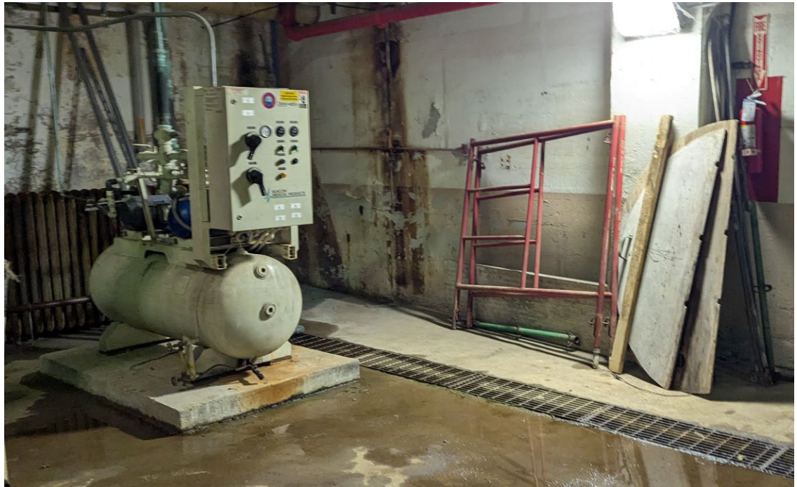
Plant #1 – Vacuum Priming System
