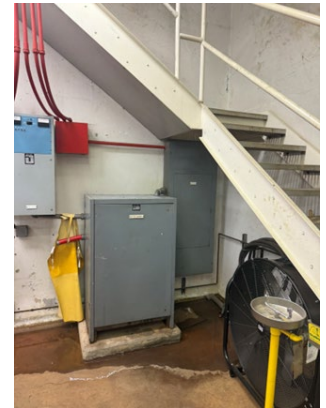
Water Pooling Around Electrical Equipment
