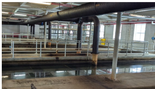
Plant #1 – Stainless Steel Air Scour Piping
