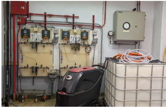
Plant #1 – Applied Water Chlorine Analyzers
