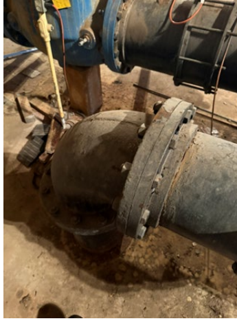
Altitude Valve Bypass Piping
