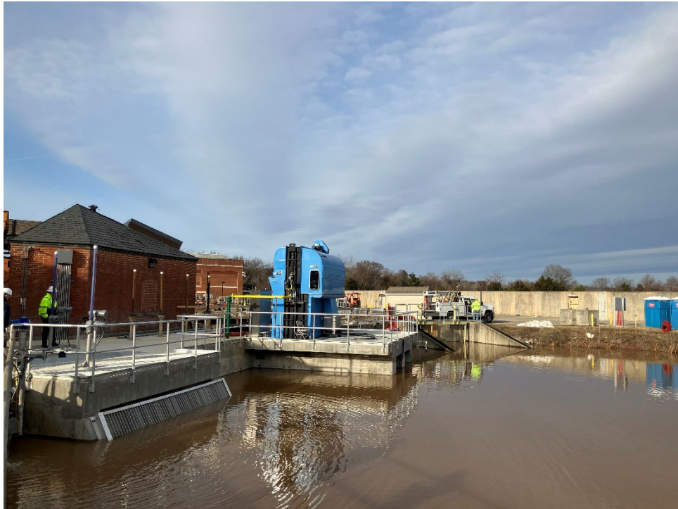
Typical Raw Water Intake. Fixed Bar Rack (Left) and Pump No. 1 Traveling Screen (Center)
