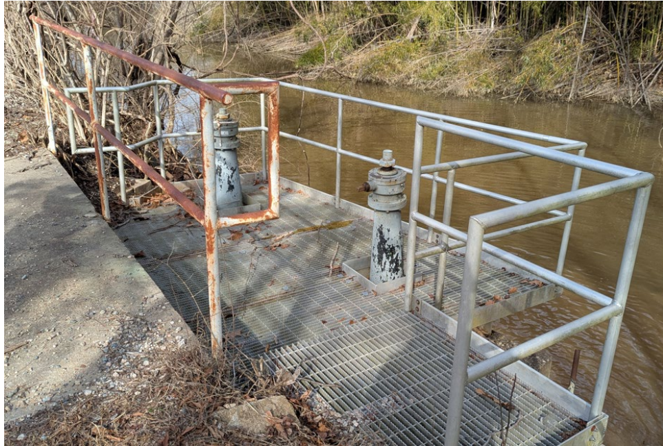
Kanawha Canal to Pre-sedimentation Basin Gate Valves
