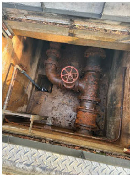
Vault with Tank Drain
