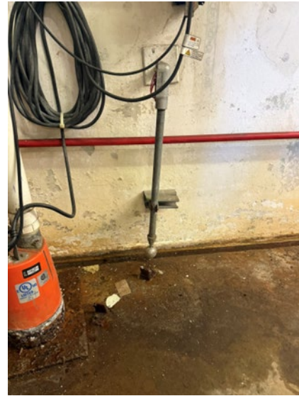
Sump Pump and Floor Flood Alarm
