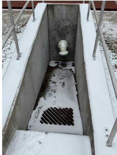
Tank Drain Discharge Structure
