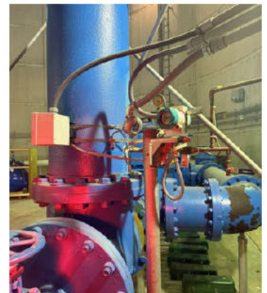
Tank Level Transmitter
