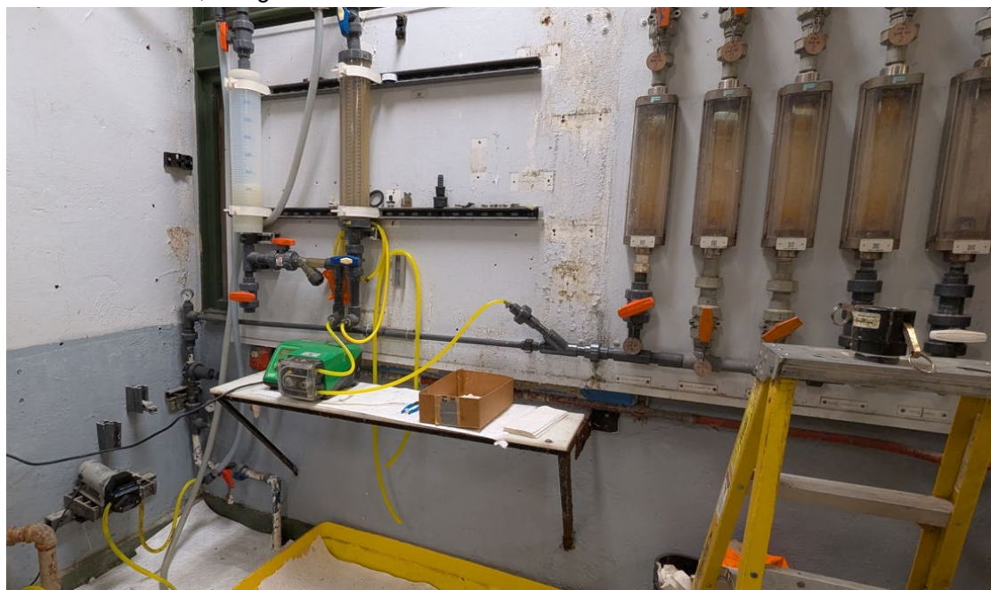
Plant #1 – Polymer Chemical Storage and Feed
