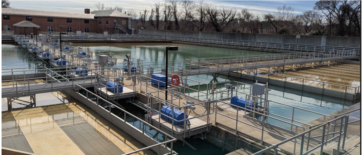
Sedimentation Basins and Plate Settlers
