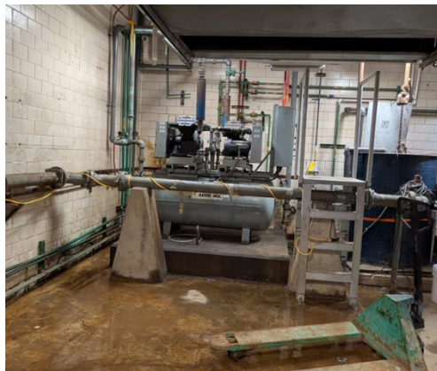
Plant #2 – Vacuum Priming System
