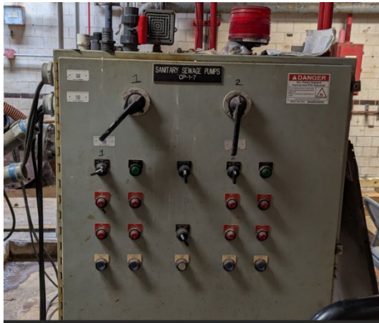
Sanitary Sewage Control Panel
