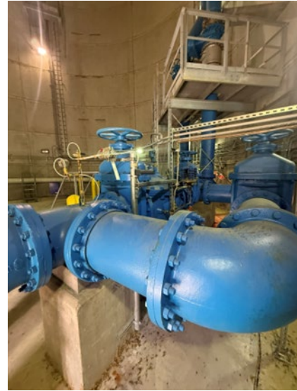
Altitude Valve and Bypass Line
