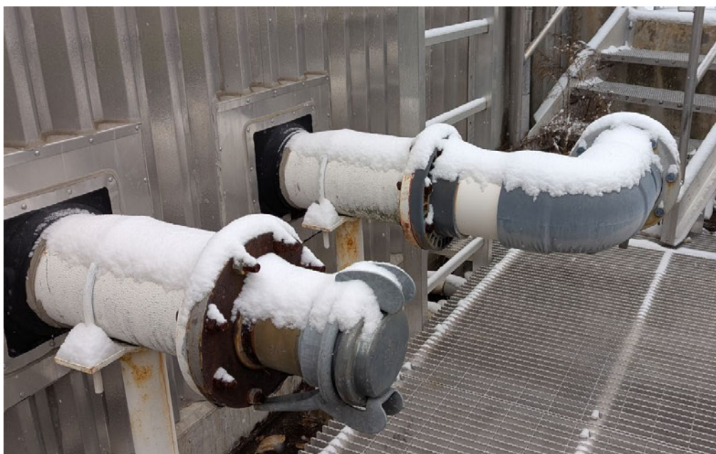
Plant #1 – Drain Suction and Discharge Connection
