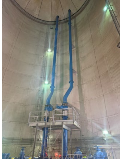
Influent and Effluent Lines
