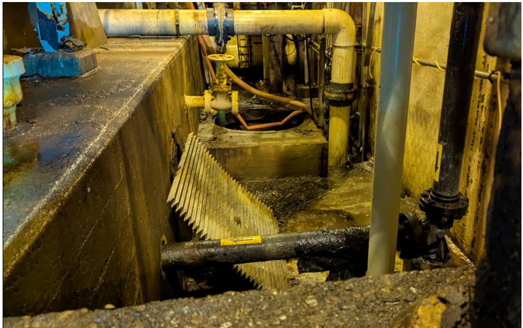
Plant #2 Piping Gallery. Sump with Permanent Dewatering Suction Pipe and Standing
