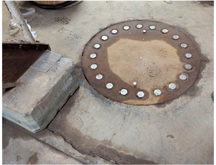
Bolted Access Hatch and Concrete Crack in Plant #2
