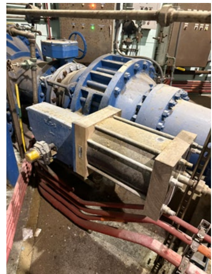
Pump Discharge Valve with Cylinder Actuator
