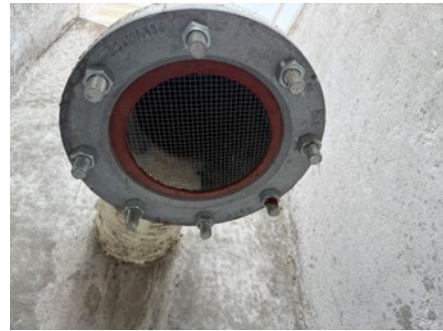
Tank Drain Discharge with Screen
