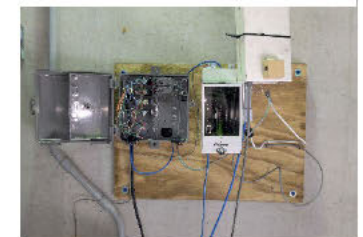
Equipment in top right of image is mounted on conduit using ziptie.
