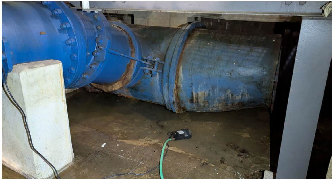
Standing Water and Temporary Sump Pump in Plant #1 – Pumping Room
