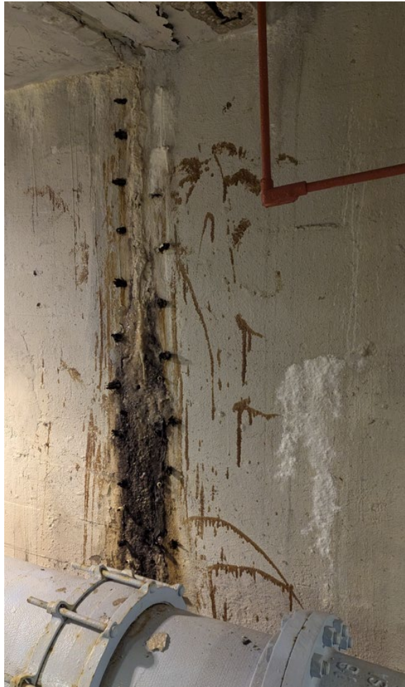
Filter 10 Wall Damage and Leaks – Plant #1
