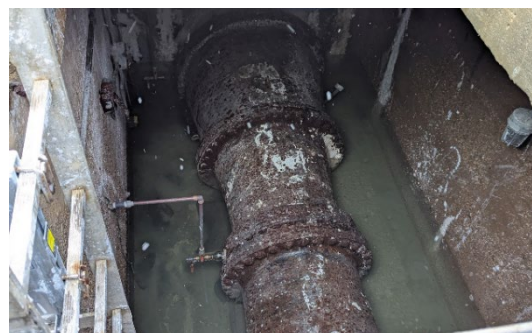
Plant #1 – Venturi Flow Meter
