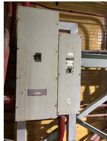
Xfmr Secondary Breaker and Limehouse Panel Breaker
