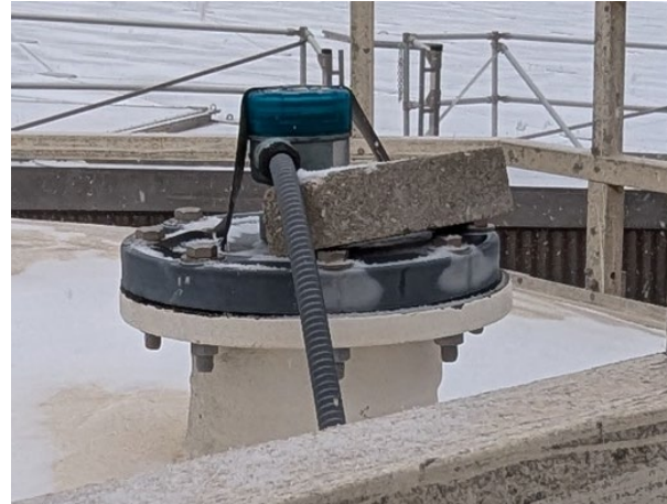
Caustic Storage Tank Level Transducer
