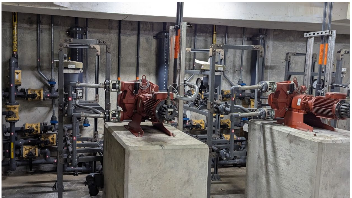
PAC Slurry Feed Pumps
