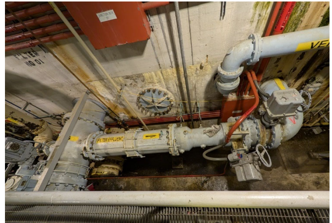
Filter Gallery Effluent Valves
