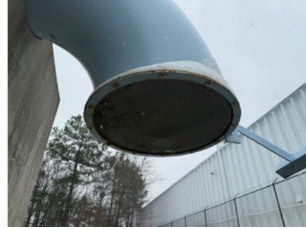
Screen Flapper Valves
