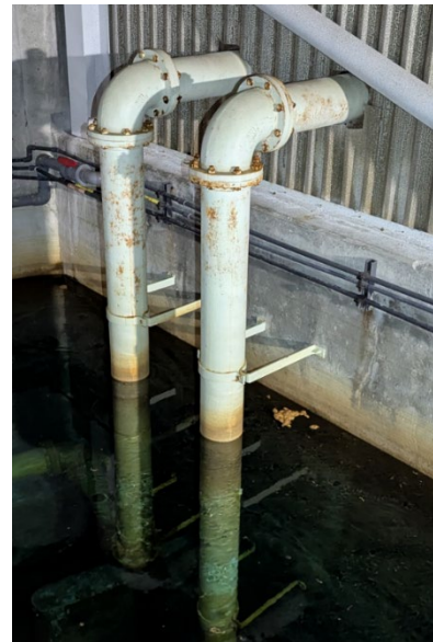
North Chlorine Contact Basin – Drain Suction and Discharge
