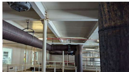
Plant #1 – Stainless Steel Air Scour Piping
