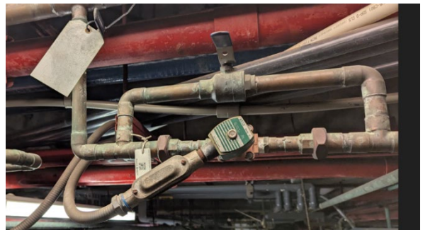
Plant #2 – Vacuum Priming Solenoid and Bypass
