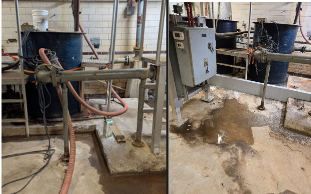
Figure 4 Containment berm around sanitary sewage tanks (Left- SEH Condition Assessment Report, Right- August 7, 2025)
