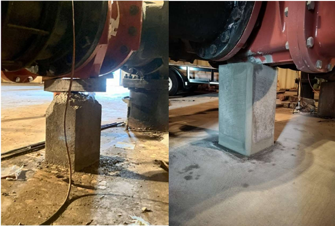
Figure 6 Warwick Road Support (Left- Sanitary Survey, Right- August 2025)
