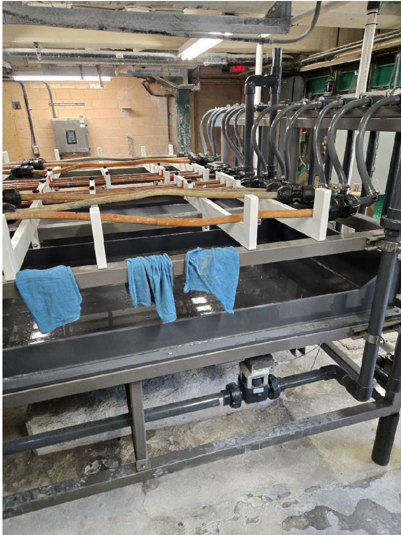
Figure 26. Pipe loop installation
