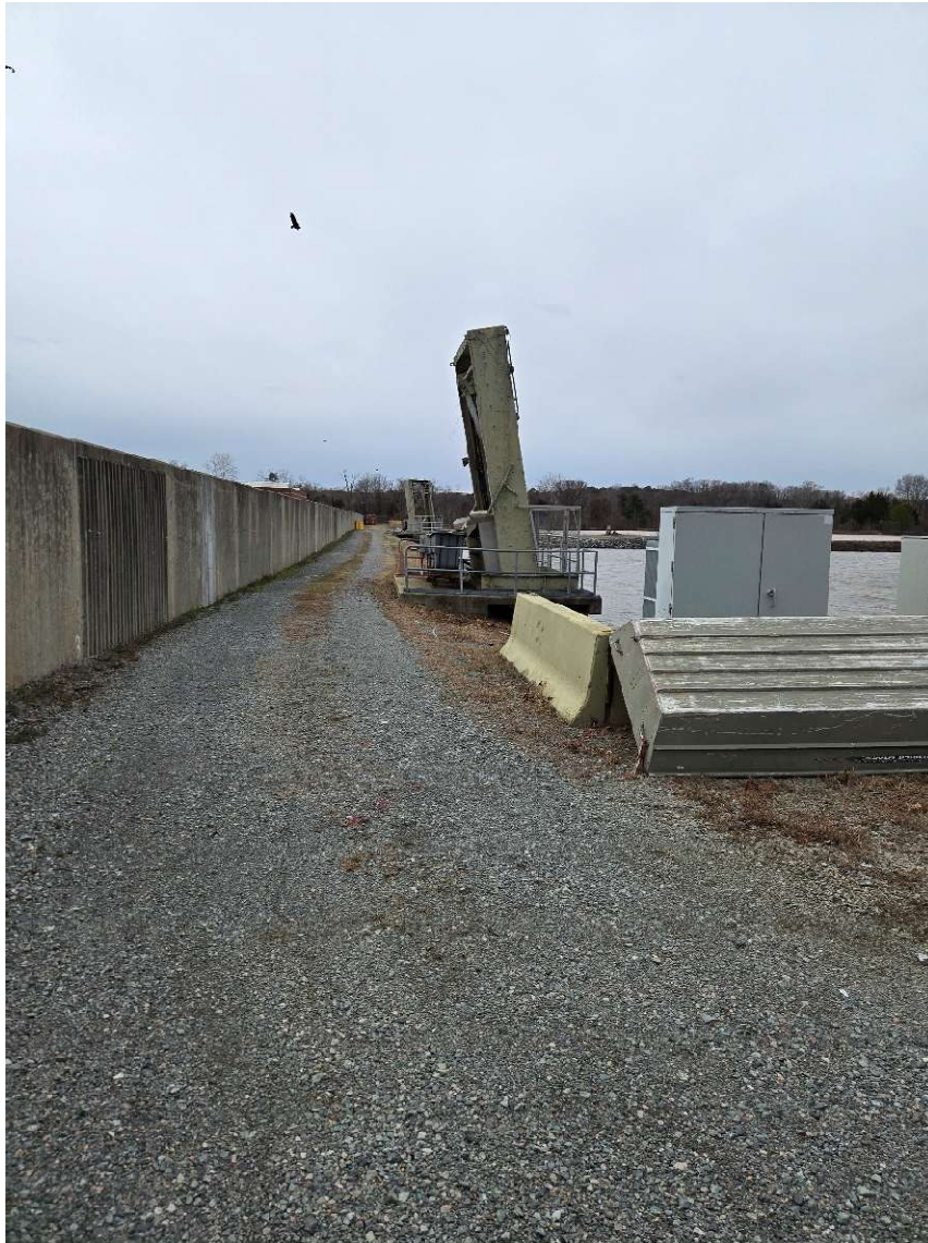
Figure 5. Pre-sed traveling screens
