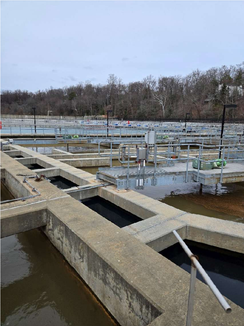
Figure 13. Flocculators
