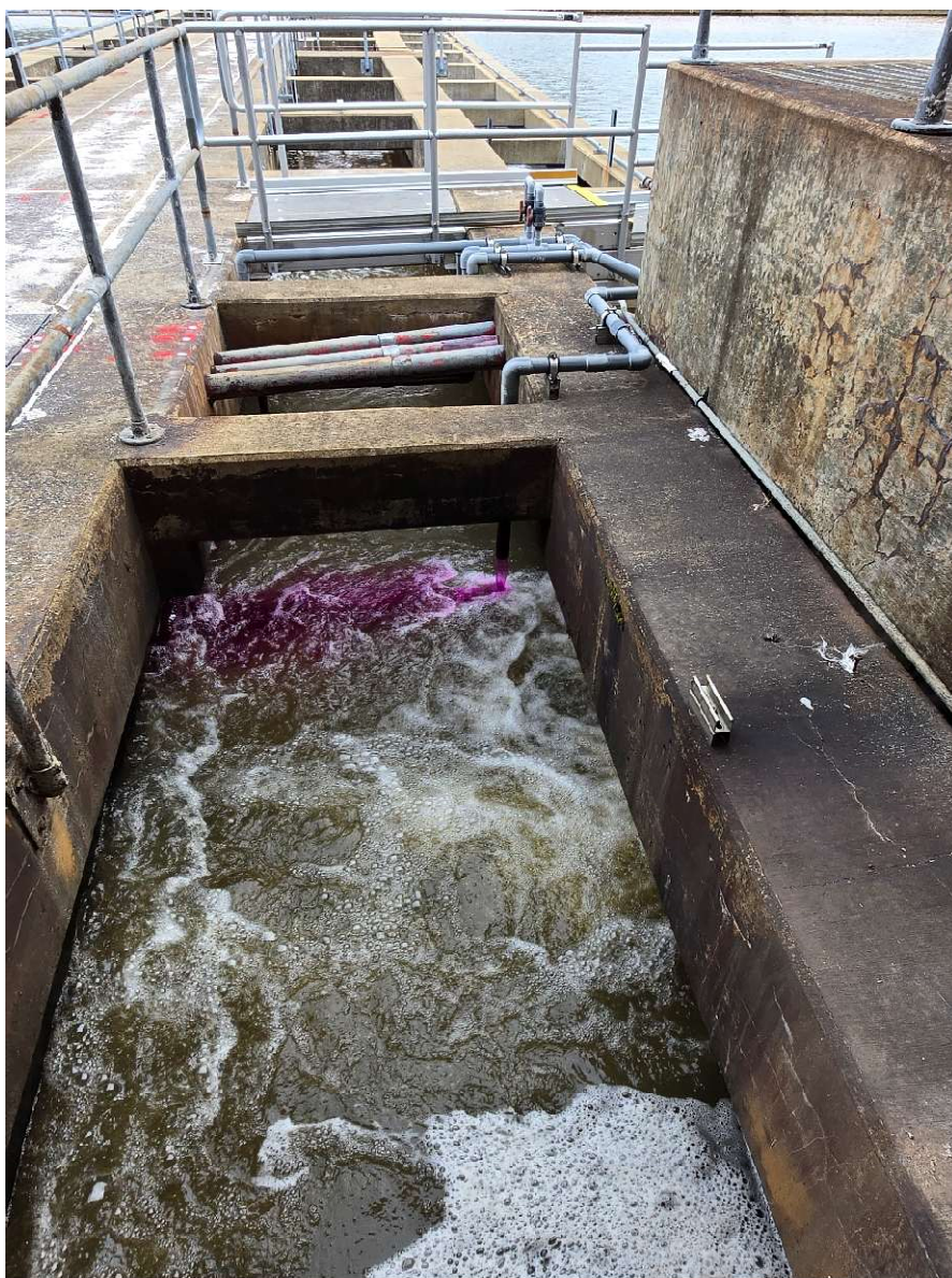
Figure 11. Permanganate feed year-round
