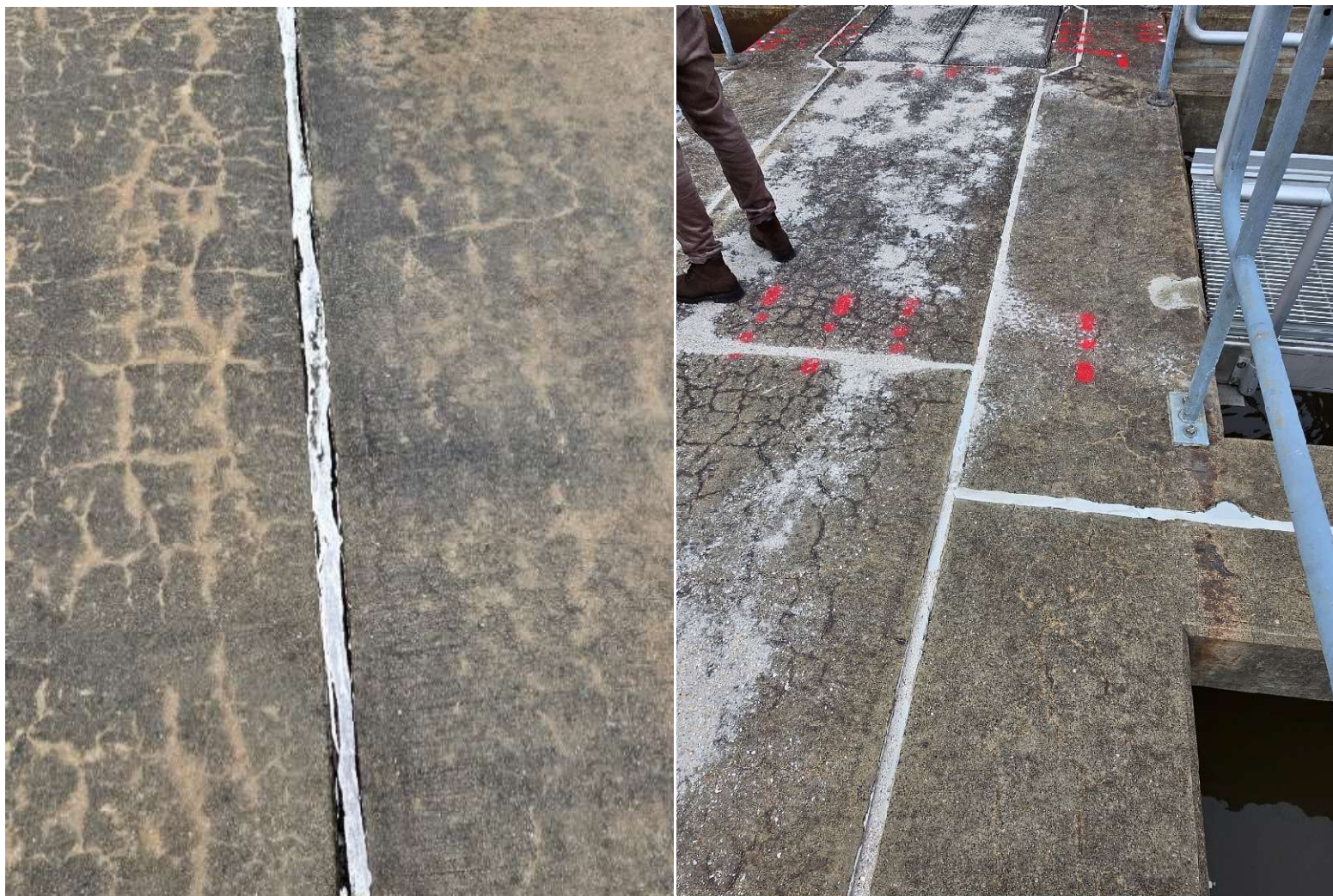
Figure 12. Sedimentation basin walkway (2025 left), sealed (2026 right)
