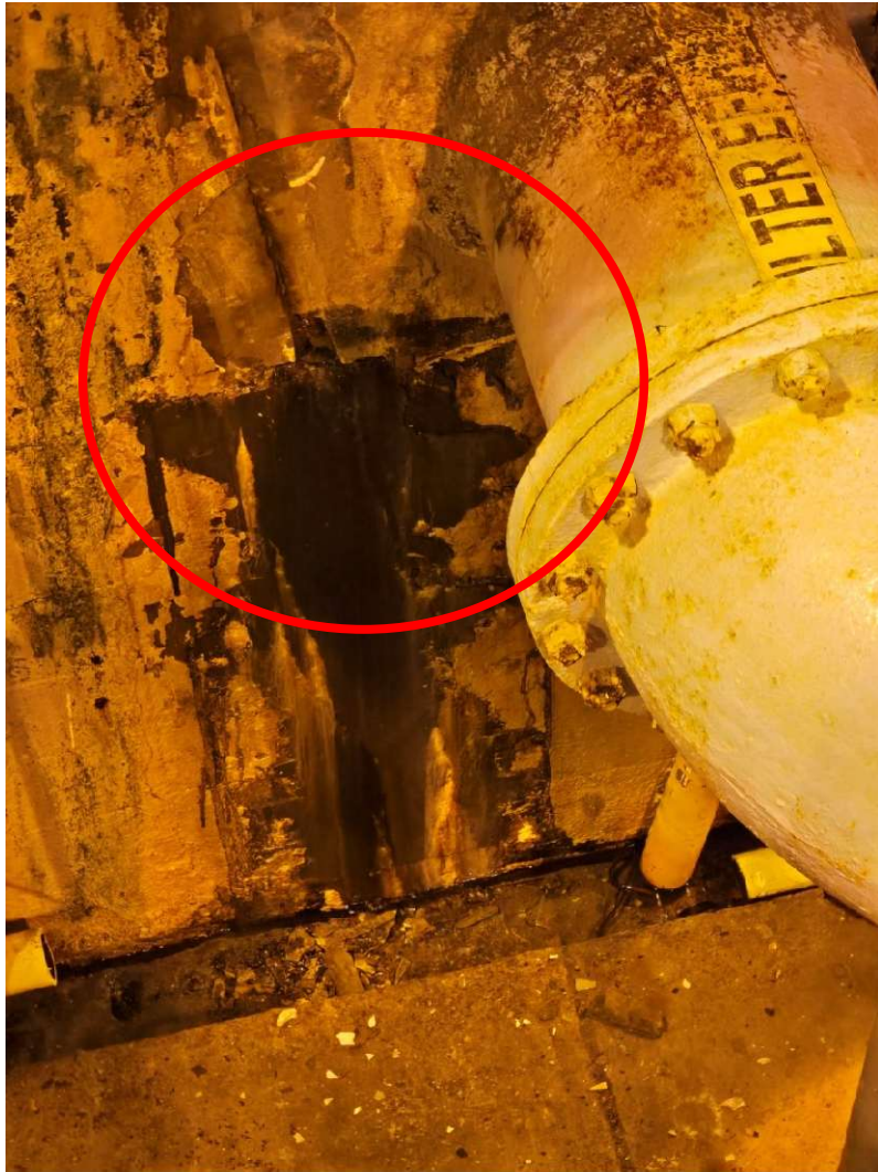
Figure 16. Filter 6 leaking through wall (2025); No leak observed (2026)
