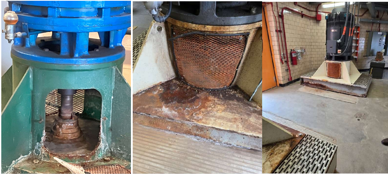
Figure 9. Raw pump motor screen (2025 left), Screen intact, all raw water pumps checked (2026 two photos on right)
