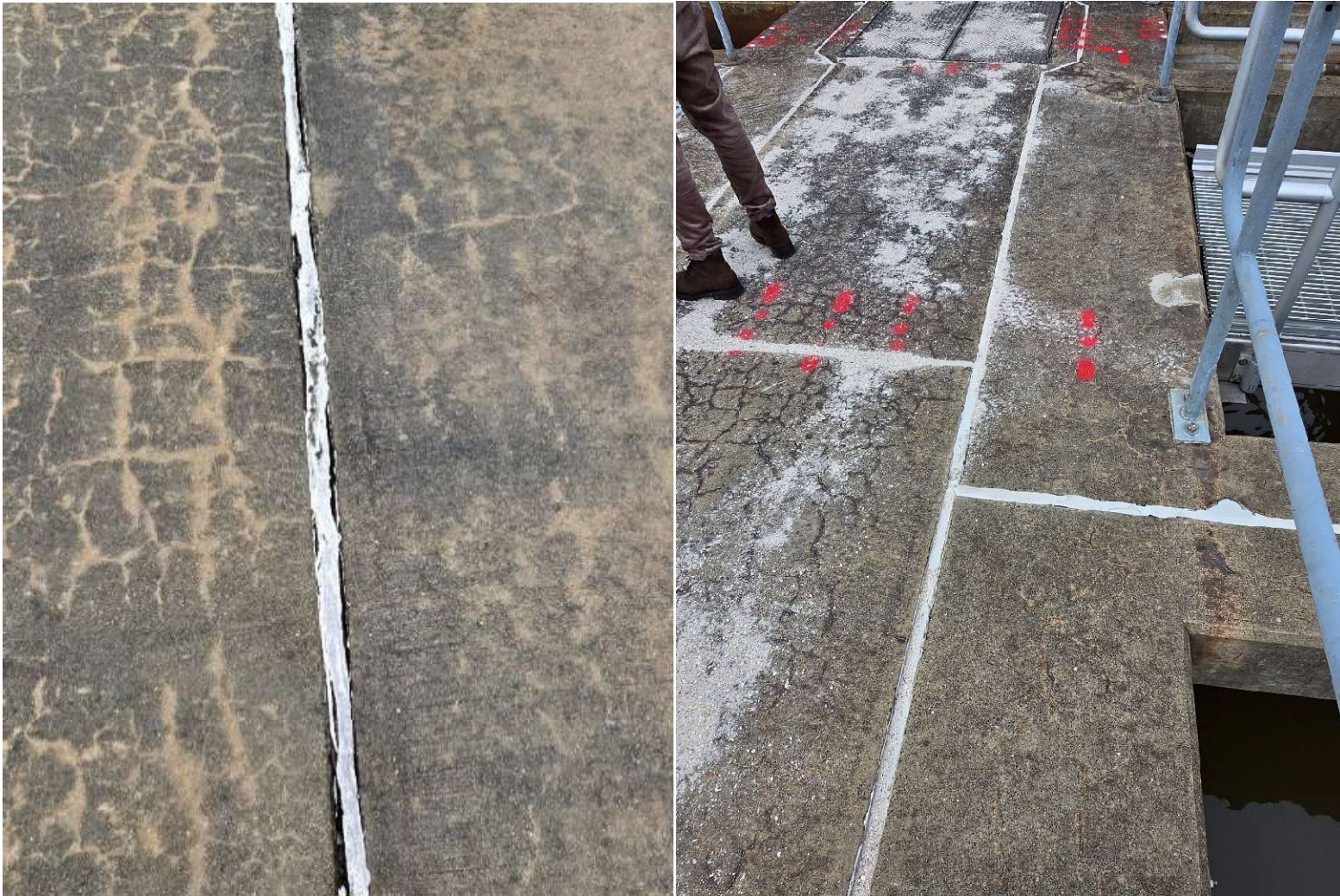
Figure 12. Sedimentation basin walkway (2025 left), sealed (2026 right)
