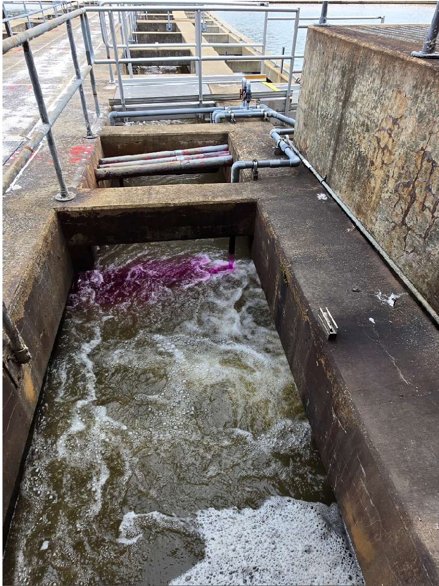
Figure 11. Permanganate feed year-round
