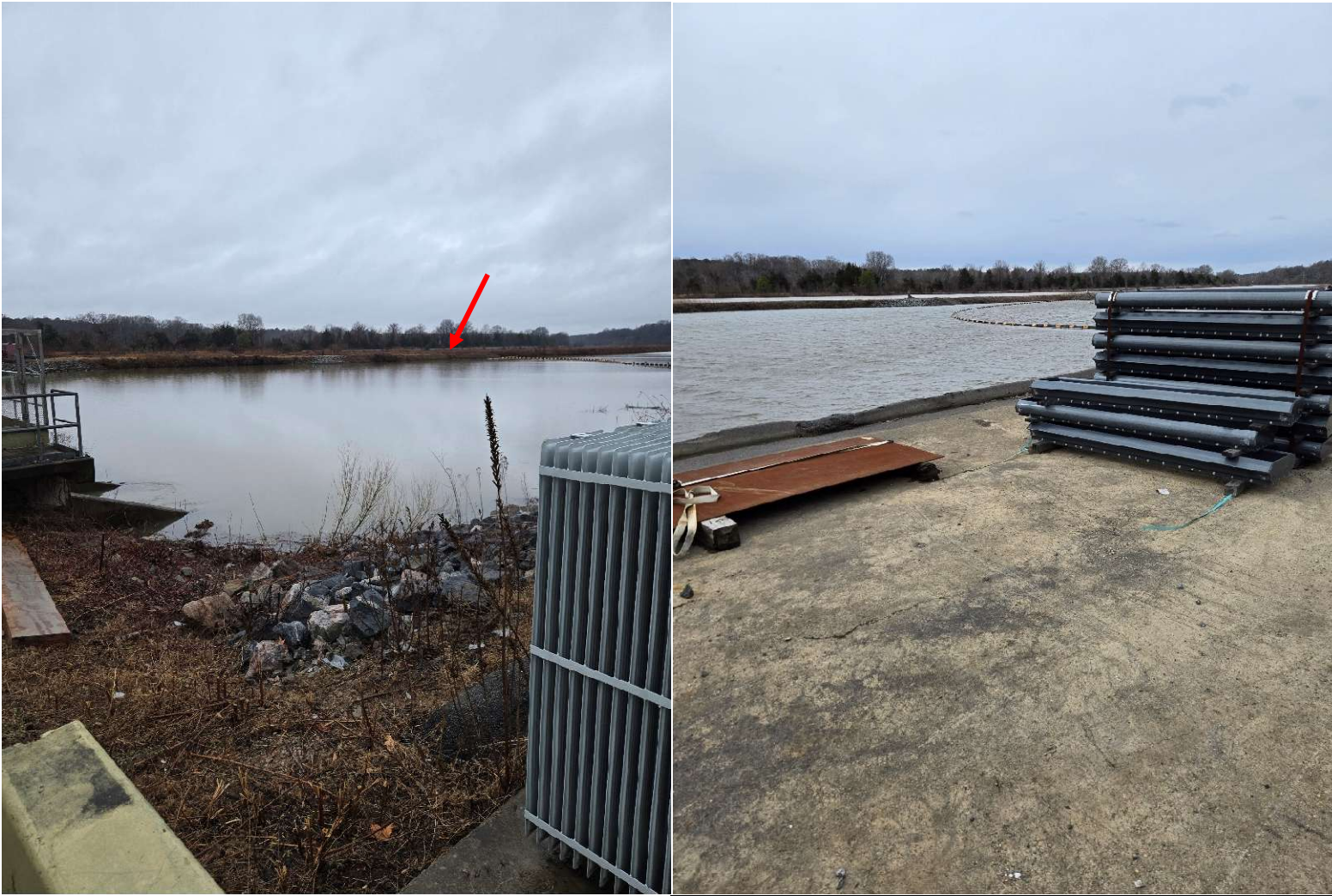
Figure 6. Earthen berm between lagoon and raw water intake channel (2025 left), Shrubs less growth observed (2026 right)
