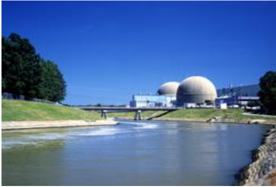
Surry Power Station
