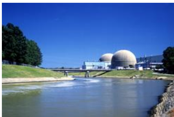
Surry Power Station
